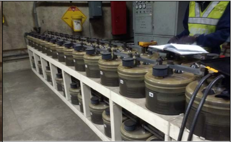
Figure 4: Measuring Round-Cell Voltage with Multimeter
