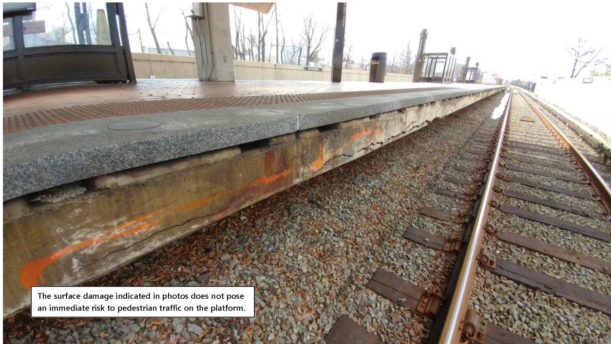
Figure 1: General condition of existing platforms (track 2 shown). Existing concrete edge is generally deteriorated.
