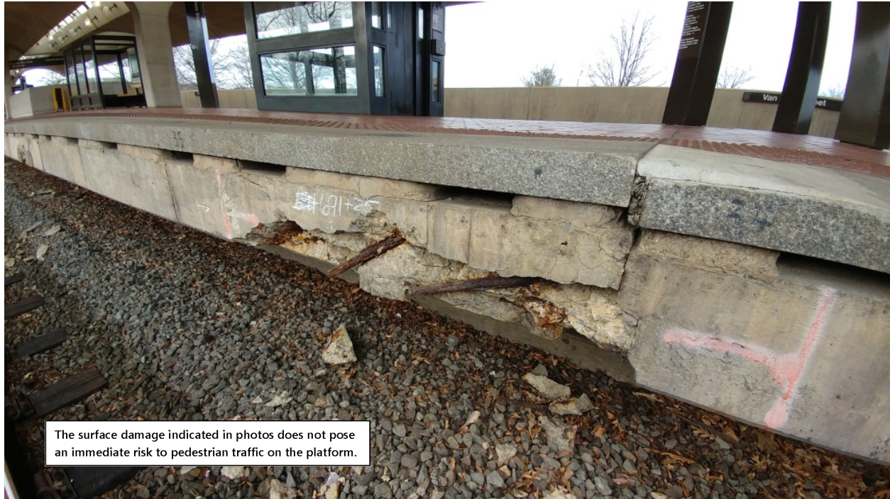
Figure 5: Large spall with exposed reinforcing steel at the edge of Track 1 platform, Chain Marker 691+25
