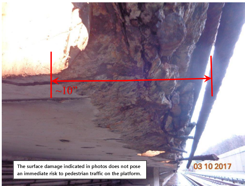
Figure 4: Close-up view from underside of platform edge. Most of spalls are within 5” from the edge of concrete. 10” is the limit for existing deterioration condition.
