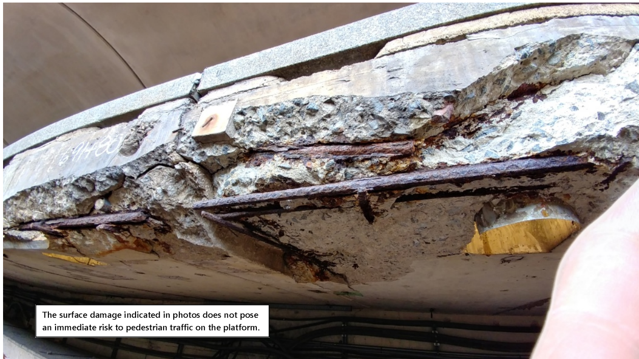
Figure 6: Large spall with exposed reinforcing steel at the edge of Track 1 platform, Chain Marker 691+90
