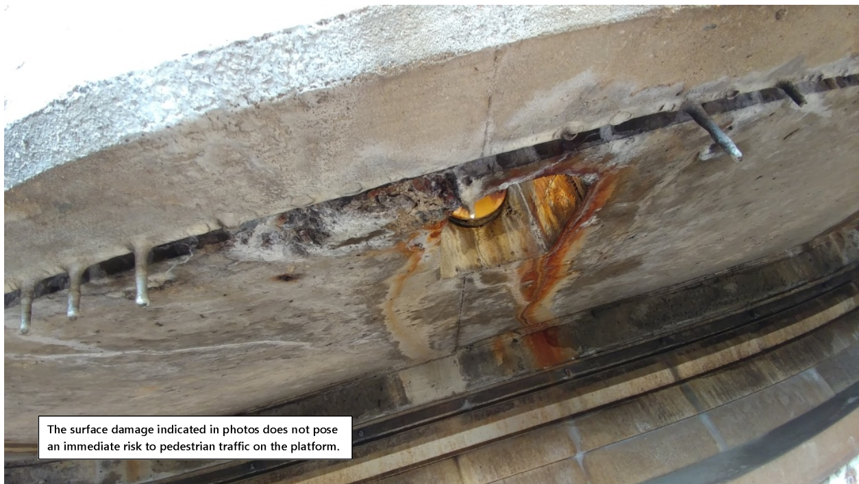
Figure 2: Typical deterioration at bottom of the slab with cracks and efflorescence near the lights
