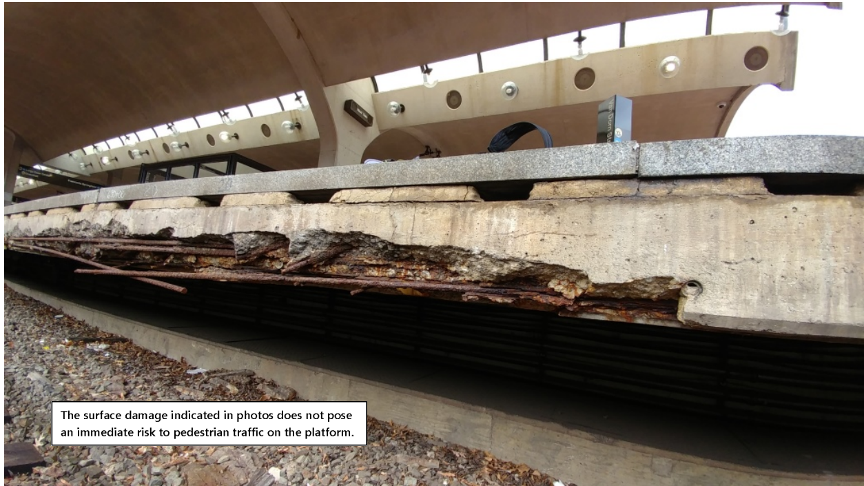
Figure 4: Large spall with exposed reinforcing steel at the edge of Track 1 platform, Chain Marker 690+00
