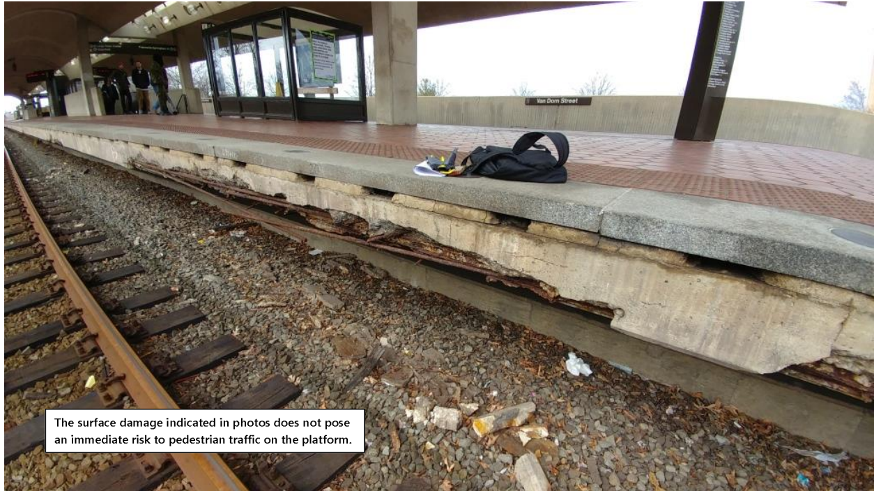
Figure 3: Large spall with exposed reinforcing steel at the edge of Track 1 platform, Chain Marker 690+00
