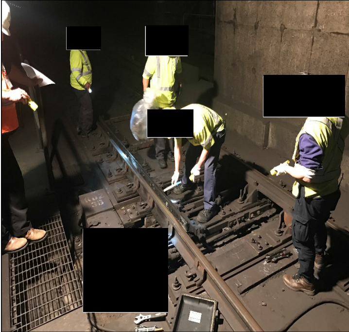
M3 Switch Machine (Mechanic Checking Point opening)
