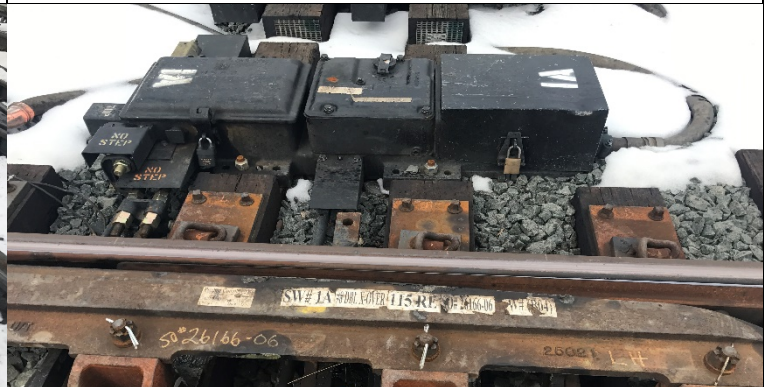
US&S M3 Electric Switch Machine
