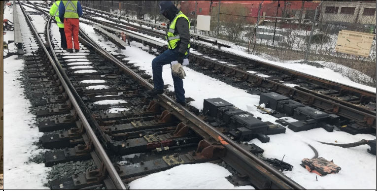
ATC Mechanic Inspecting Switch Machine Area
