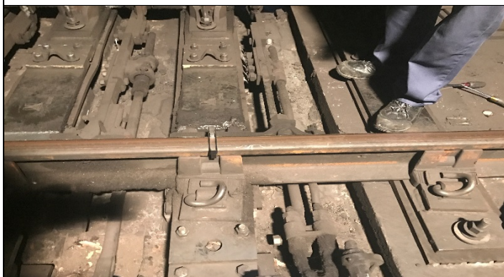
1/4 Inch Obstruction Gauge in Reverse Point
