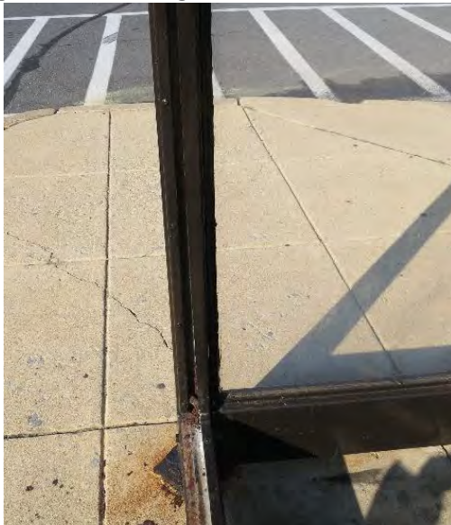
Figure 103: Frame Rust, Shelter D
