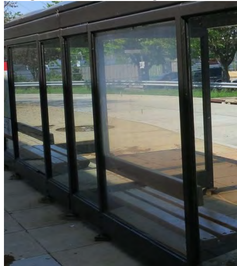
Figure 69: Panel Fading, Shelter D
