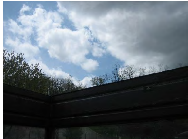
Figure 76: Missing Dome Top, Shelter C
