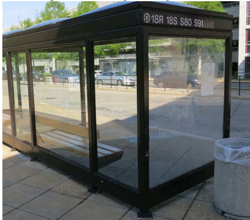
Figure 81: Panel Fading and Damage, Shelter D
