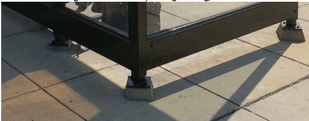
Figure 173: Minor Pad/Footing Cracking, Shelter A
