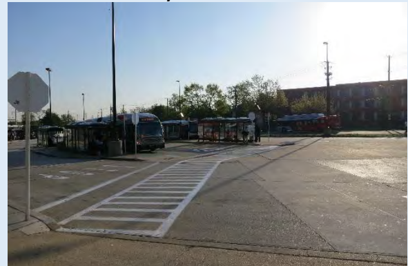
J-K Bus Bay Platform South End
