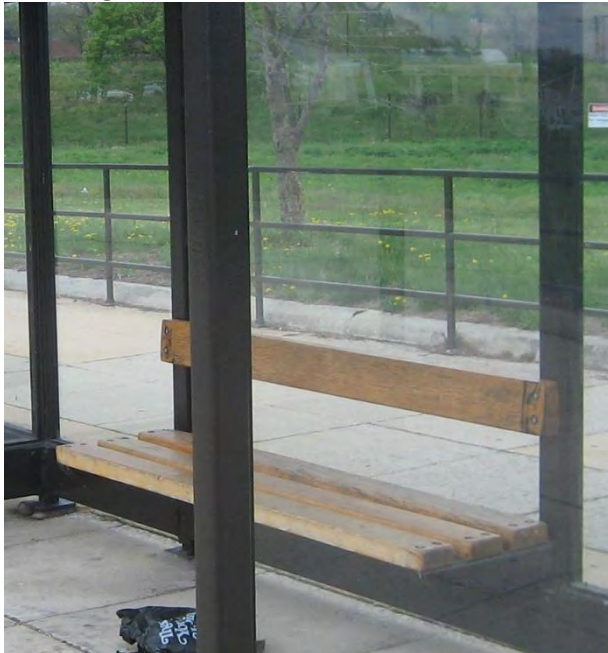
Figure 186: Wear on Bench, Shelter A
