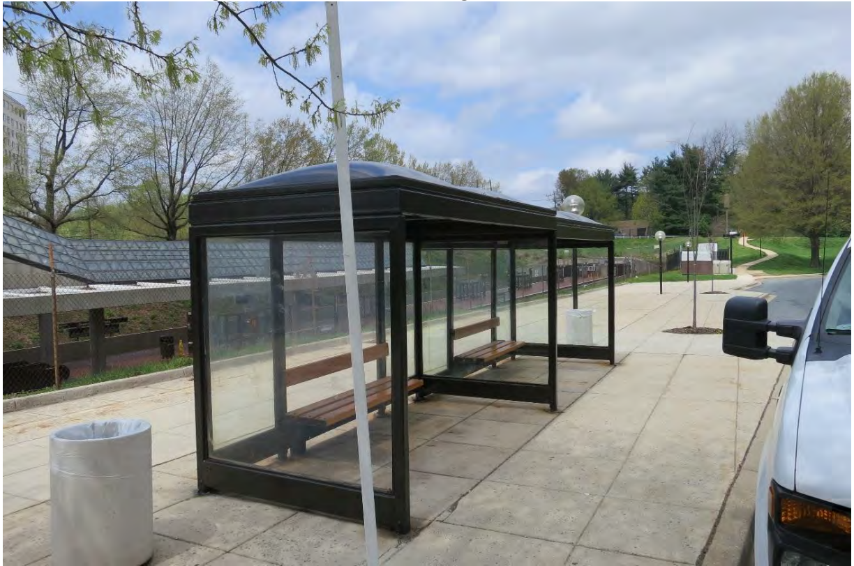
Figure 91: Overall Above Average Condition, Shelter D
