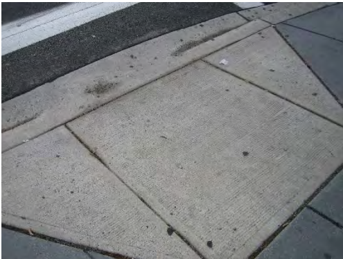
Figure 116: Curb Ramp at Northwest Corner
