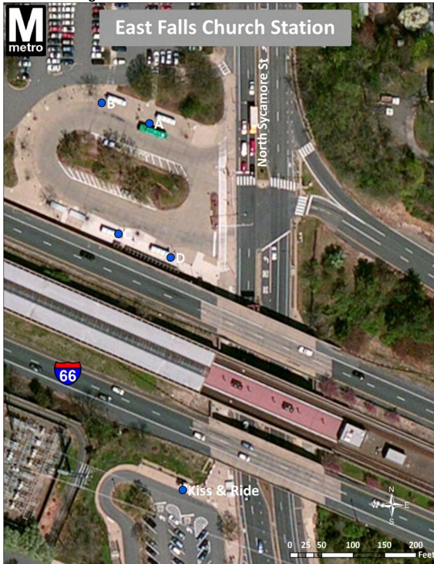
Figure 60: East Falls Church Station Bus Shelters
