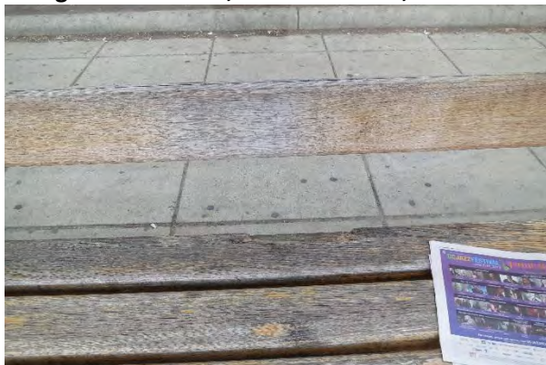
Figure 191: Worn, Cracked Bench, Shelter B
