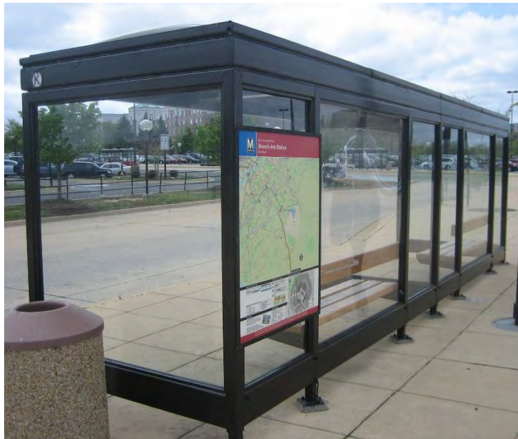
Figure 32: Good Overall Shelter Condition, Shelter K
