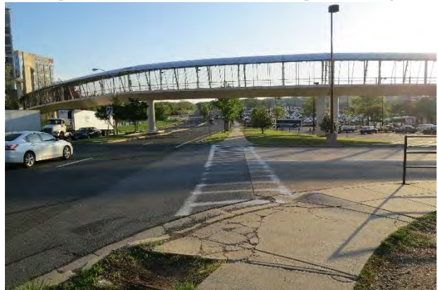
Figure 74: Crosswalk Traversing Driveway
