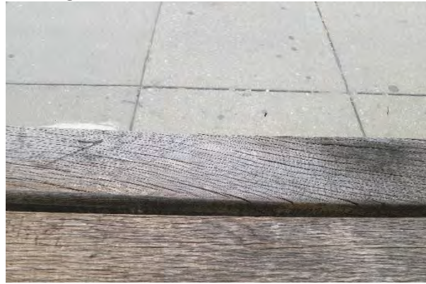
Figure 28: Weathered Bench, Shelter B
