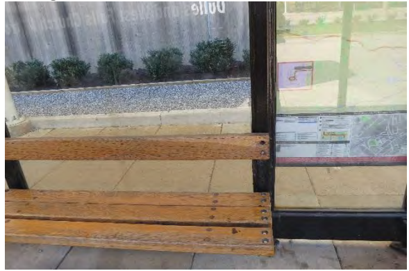
Figure 179: Frame Rust, E South
