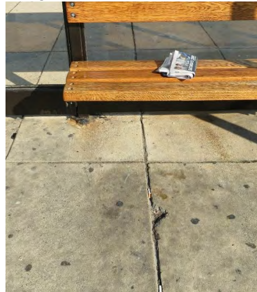
Figure 103: Frame Rust, Shelter D
