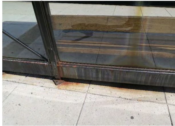
Figure 63: Faded/Scratched Panels, Kiss & Ride Shelter
