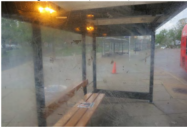
Figure 41: Smearred/Faded Panel, Shelter C
