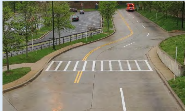
Crosswalk Traversing Central Ave Entrance Driveway
