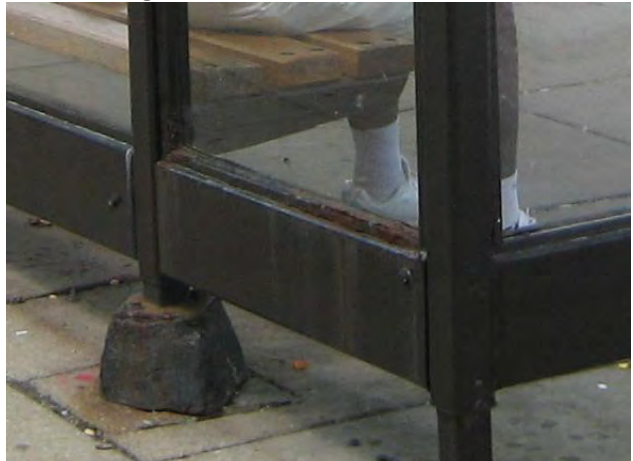
Figure 76: Missing Dome Top, Shelter C
