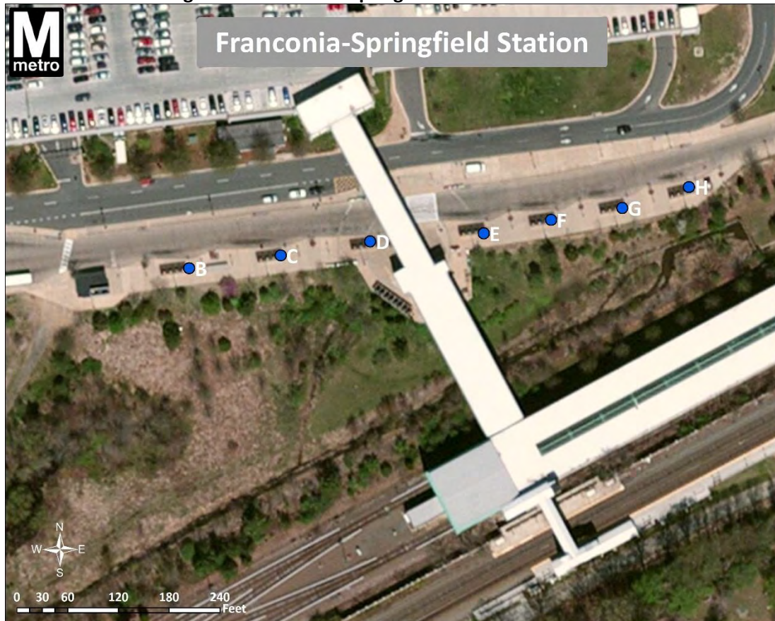
Figure 78: Franconia-Springfield Station Bus Shelters
