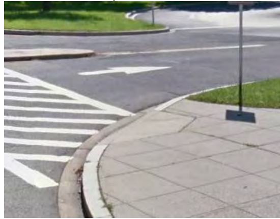
Curb Ramp at Eastern Avenue
