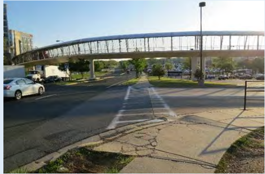
Southeast Curb Ramp at Busway/Kiss-and-Ride Entrance
