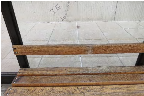
Figure 148: Worn/Damaged Bench, Shelter K
