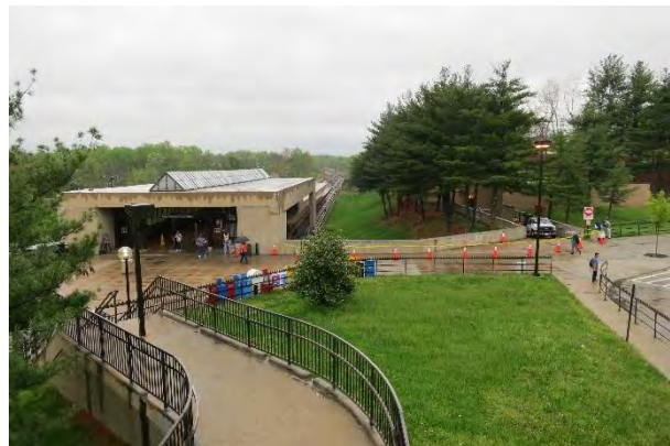
Figure 18: Stairwell from Pedestrian Overpass Down to Station Level
