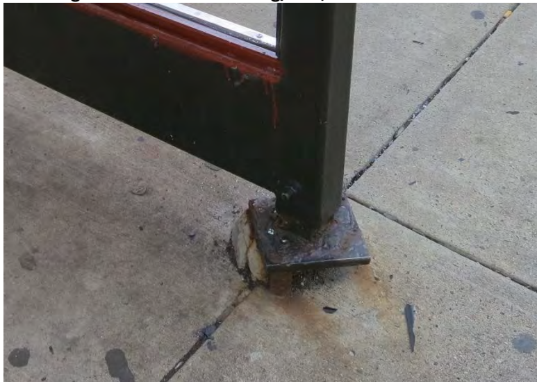
Figure 98: Cracked Footing/Pad, Kiss & Ride Shelter
