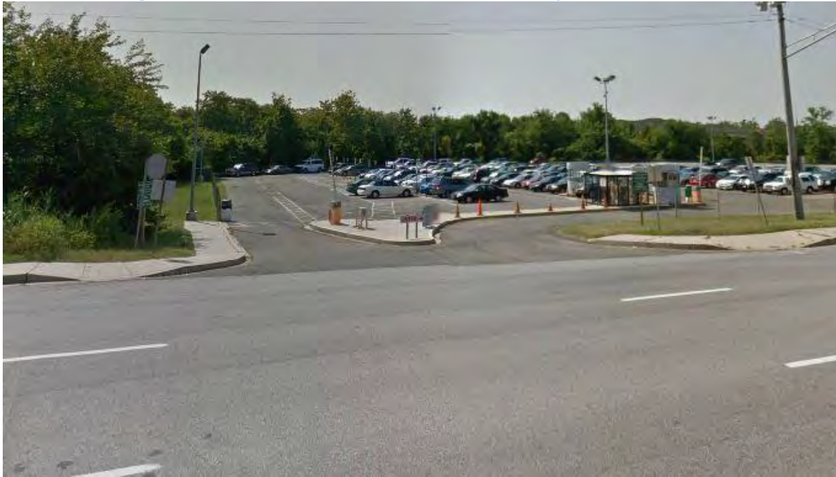
Figure 108: East Park-and-Ride (Amtrak)/Garden City Drive Intersection
