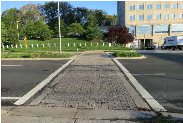
Figure 73: Crosswalk Traversing Ellin Road
