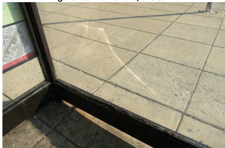
Figure 103: Frame Rust, Shelter D
