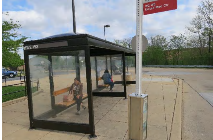
Figure 52: Smeared Panel, Good Frame Condition, Shelter C
