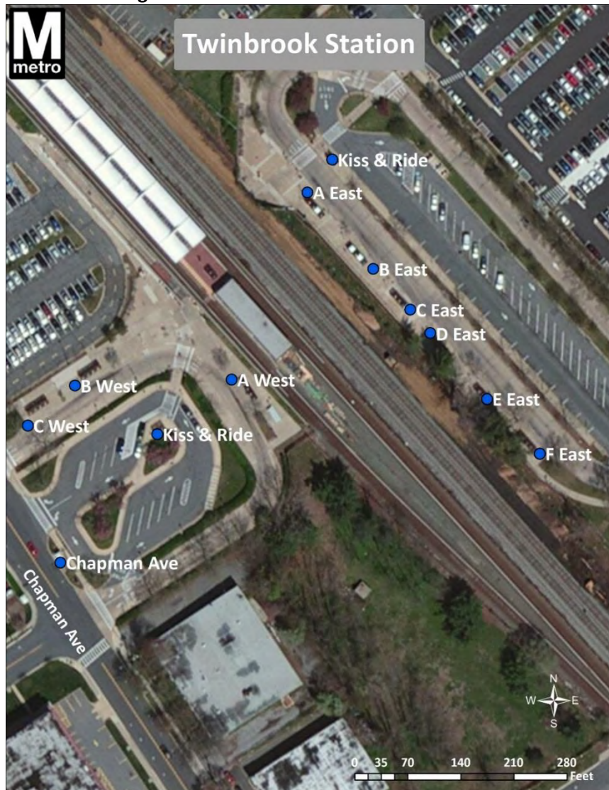
Figure 164: Twinbrook Station Bus Shelters
