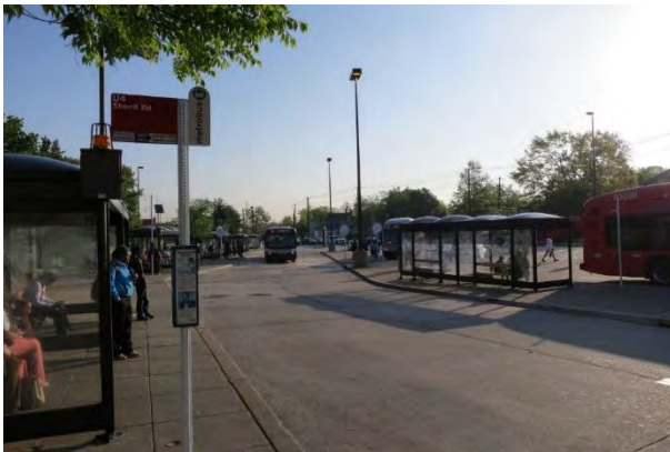
Figure 55: West Busway From Bus Bay E
