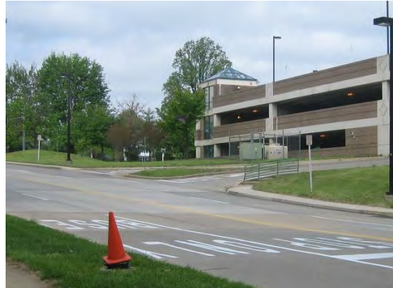
Entrance on Addison Road Entrance Driveway
