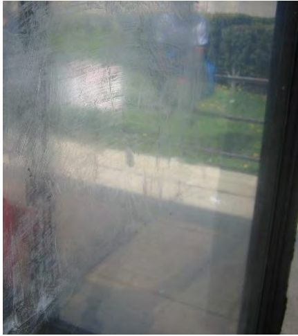
Figure 45: Smeard/Scratched Panel, Shelter E
