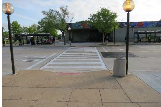
Crosswalk Between A-E Bus Bays and Metrorail Station Entrance
