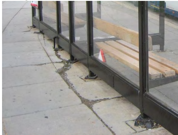
Figure 75: Poor Pad Condition, Shelter A
