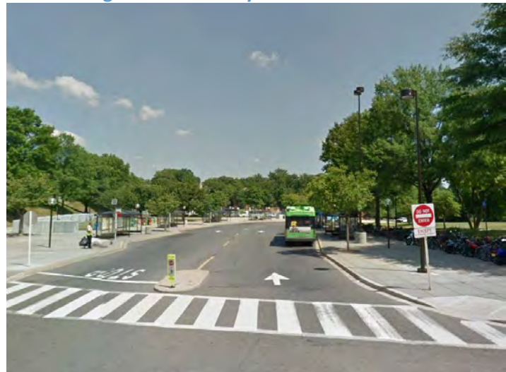
Figure 117: Busway from Cedar Street
