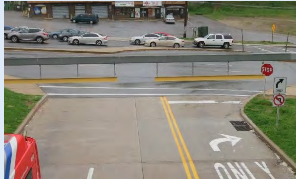
Crosswalk Traversing Central Ave Entrance Driveway
