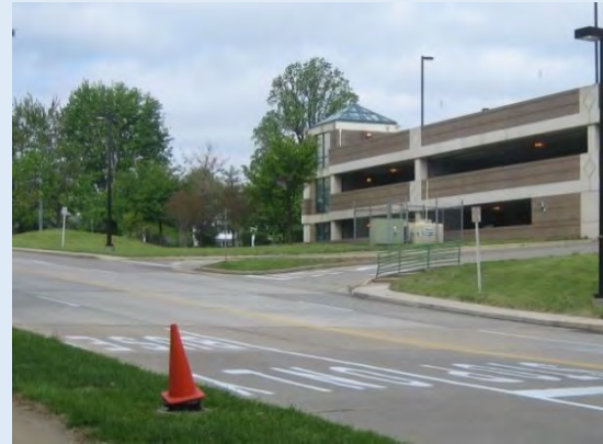
Park-and-Ride Garage Driveway
