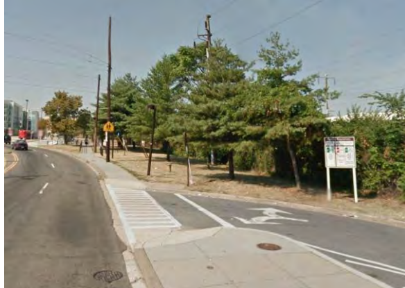
Figure 62: Kiss-and-Ride South Exit & Lack of Stop Sign
