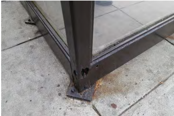
Figure 130: Hole in Frame, Shelter C
