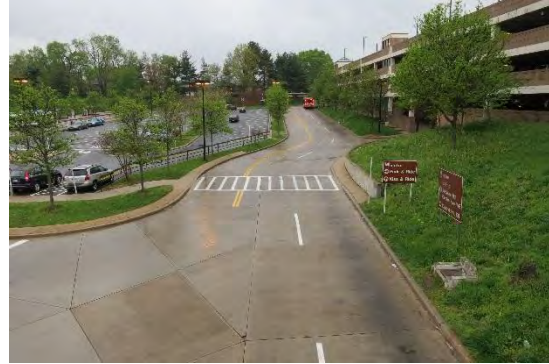
Crosswalk Traversing Central Ave Entrance Driveway
