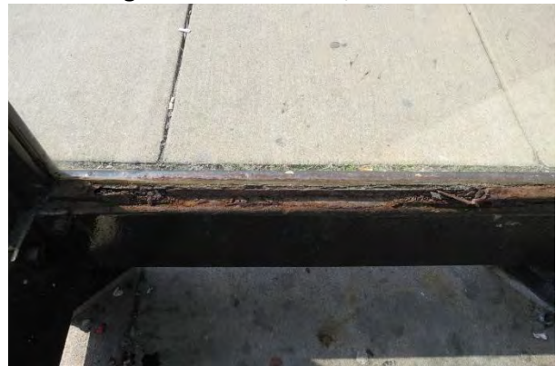
Figure 81: Panel Fading and Damage, Shelter D
