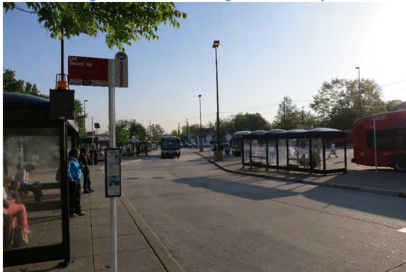
Figure 68: Lack of Fencing Behind Bus Bays
