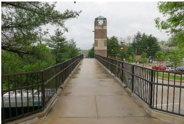
Figure 17: Pedestrian Overpass from Park-and-Ride Garage Looking East Towards Station Entrance
