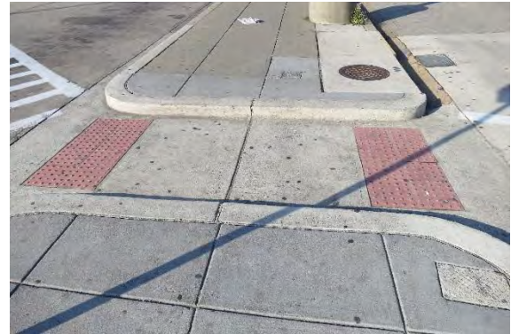
J-K Bus Bay Platform Cut-Through
