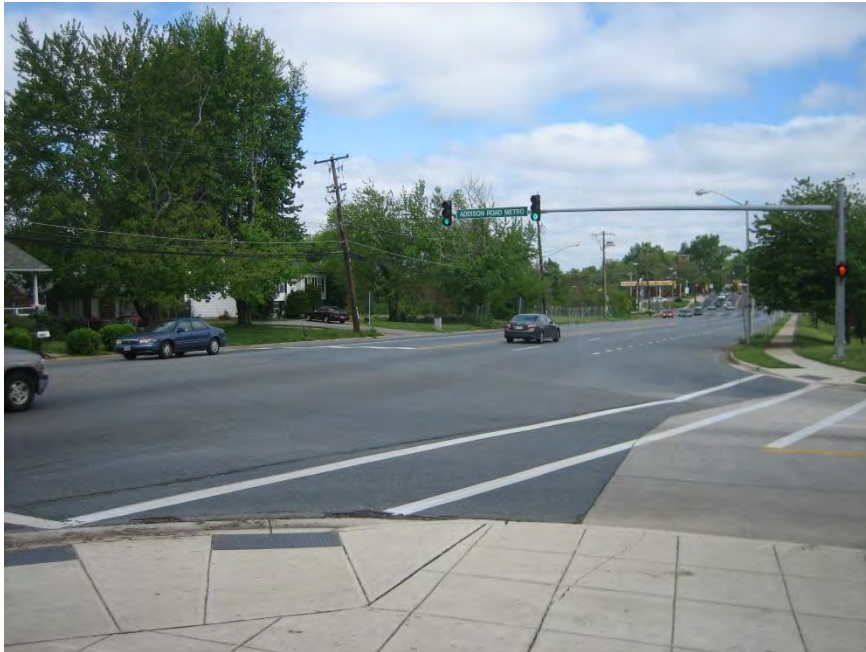
Figure 6: Addison Road Entrance Looking North
