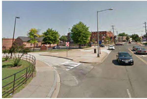
Figure 34: Martin Luther King Jr. Avenue Driveway Looking North
