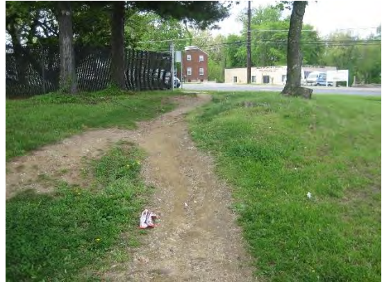
Southeast Corner of Addison Road Intersection Pedestrian Path
