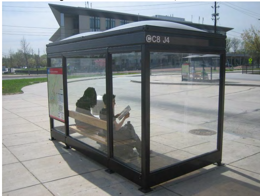
Figure 44: Good Overall Condition, Shelter C
