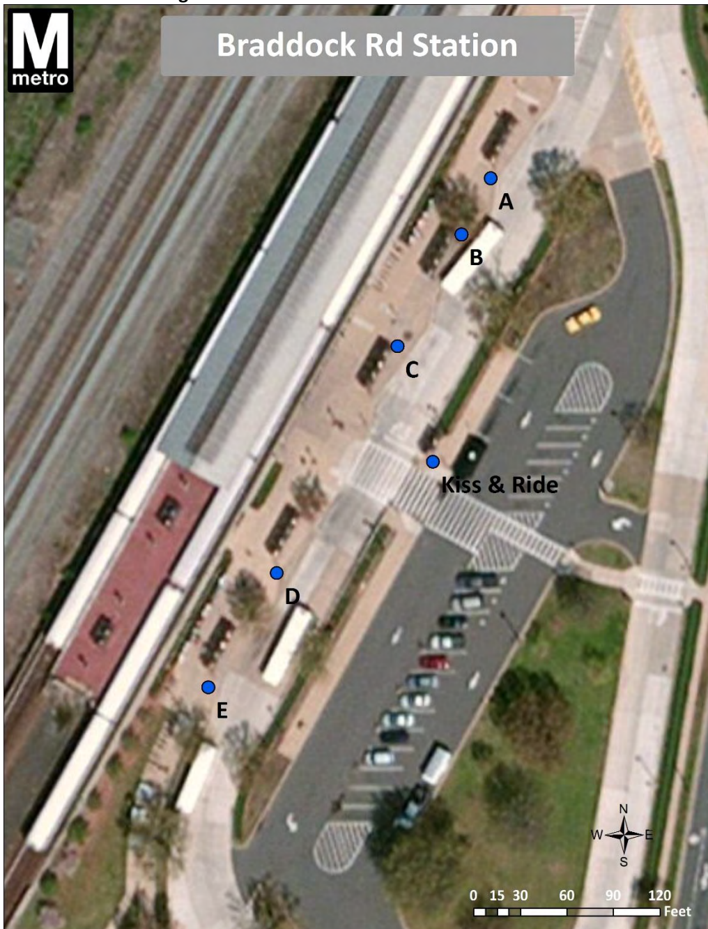
Figure 19: Braddock Road Station Bus Shelters
