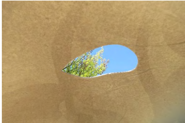
Figure 180: Hole in Dome Top, Shelter G South
