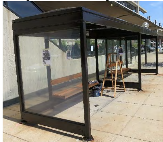
Figure 67: Frame Painting, Shelter A
