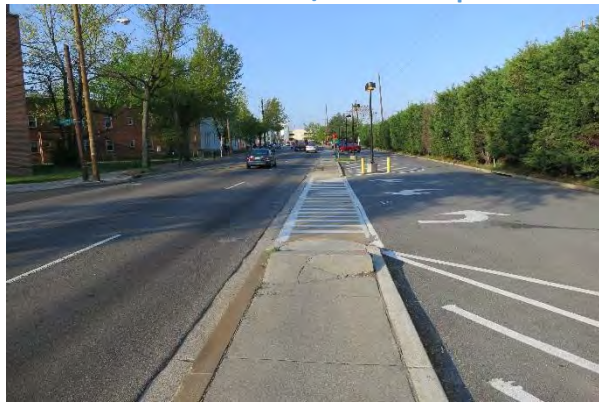
Figure 60: Kiss-and-Ride Center Entrance/Exit & Poor Sidewalk Condition/Lack of Stop Controls
