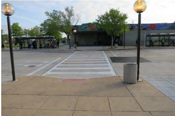
Figure 36: Main Busway and Crosswalk
