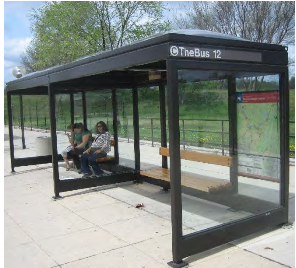
Figure 187: Good Frame Condition, Shelter C
