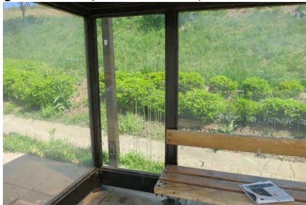
Figure 63: Faded/Scratched Panels, Kiss & Ride Shelter
