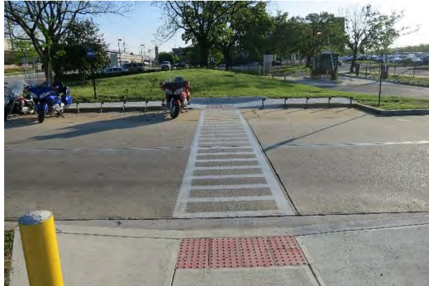
Figure 103: Egress Driveway Crosswalk at Motorcycle Parking Area
