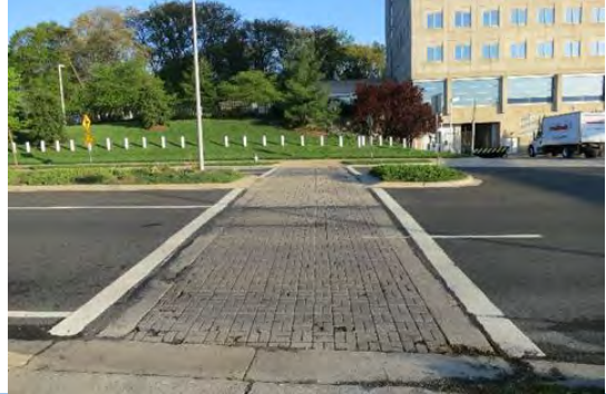
Curb Ramps at Busway/Kiss-and-Ride Entrance
