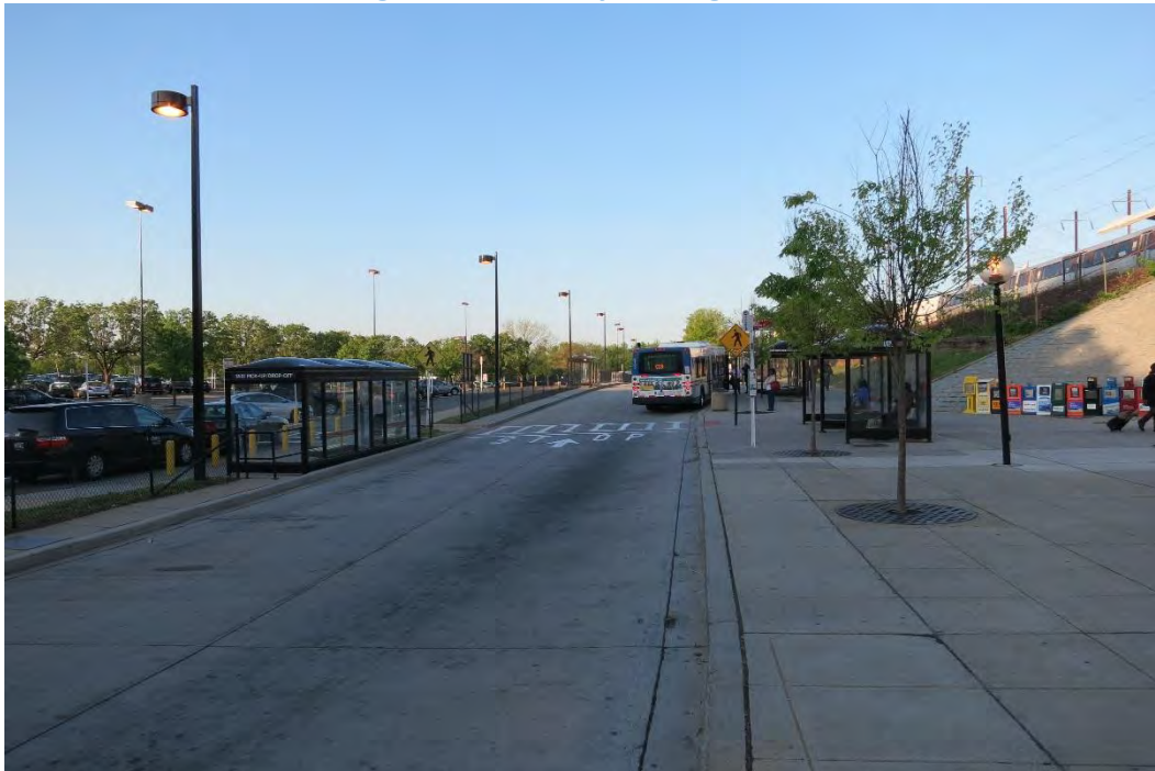
Figure 111: Busway Looking South
