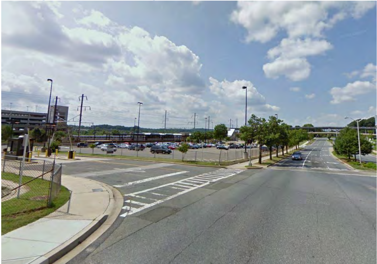
Figure 80: Park-and-Ride Parking Area Entrance on Ellin Road, West Side of Station
