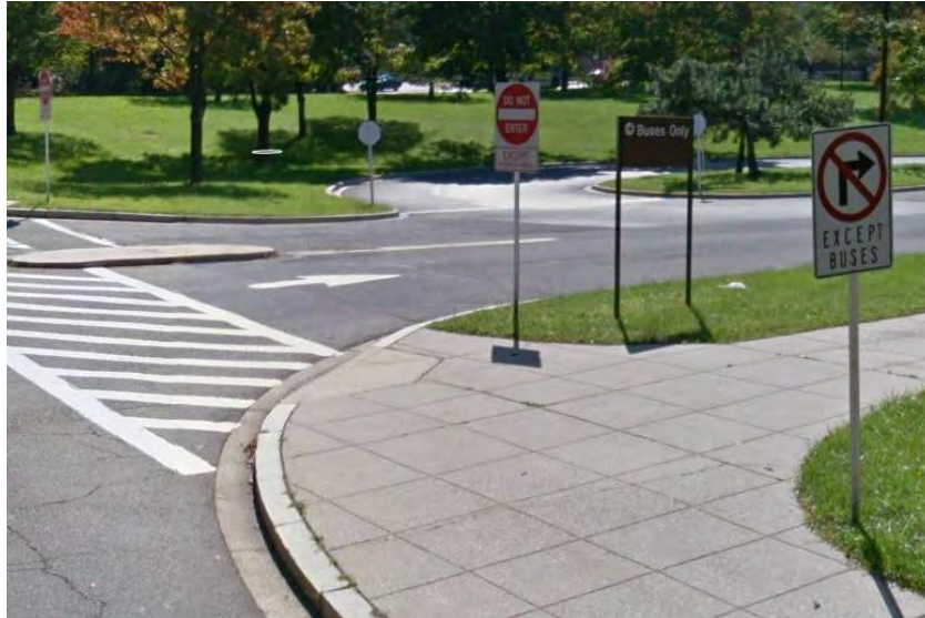
Figure 118: Eastern Avenue Southbound Signage at Busway
