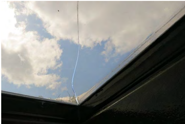
Figure 155: Cracked Dome Top, Shelter C
