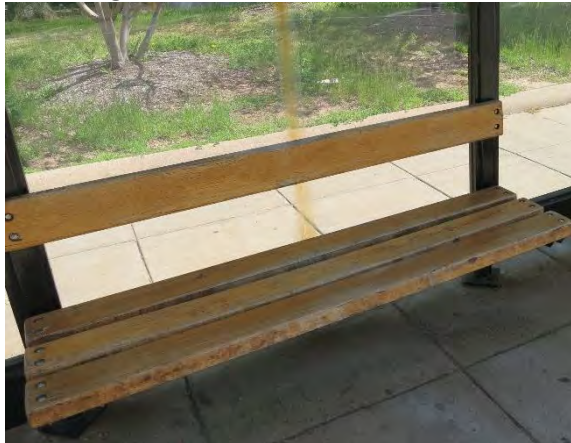
Figure 63: Faded/Scratched Panels, Kiss & Ride Shelter
