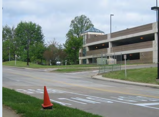
Entrance on Addison Road Entrance Driveway
