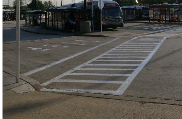
Southwest Curb Ramp on A-H Platform
