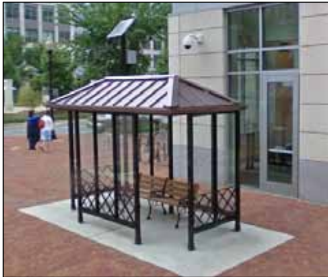
Figure 3-7 Example of Shelter Lighting Powered by Solar energy
