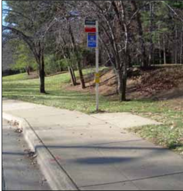
Figure 3-10 Landing Pad with Sidewalk Adjacent to Curb
