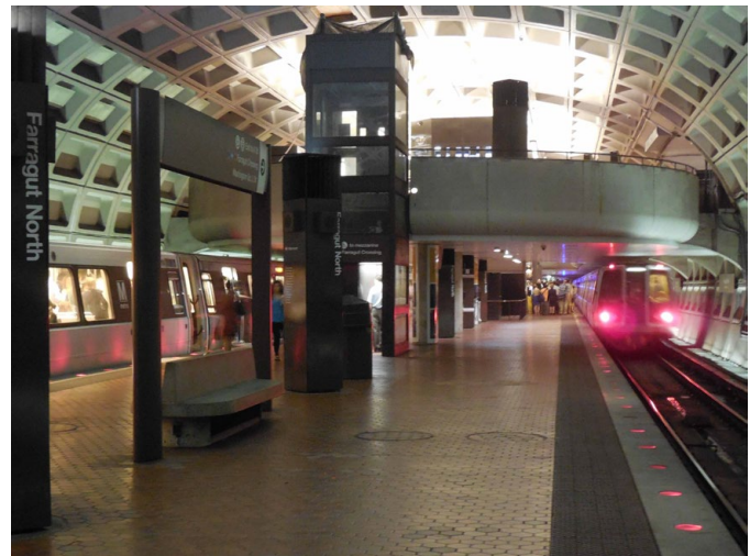
South end of platform looking towards the South Mezzanine
