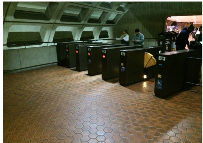
Farragut West Station, West Mezzanine, current location of ADA faregate proposed to be relocated to opposite side of station kiosk and replaced with a standard faregate to better accommodate passenger flow
