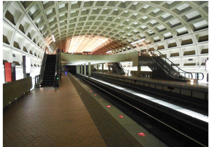
Farragut West Station, platform escalators, existing condition
