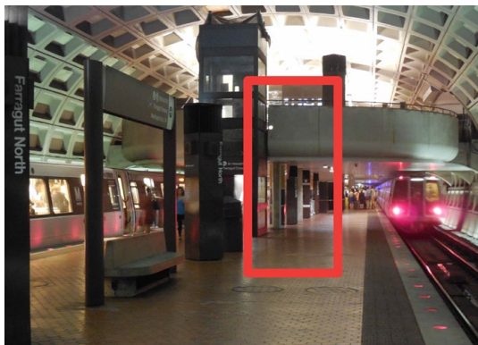
Farragut North Station, South Mezzanine proposed location of new stair; a second street elevator is also proposed at the South Entrance
