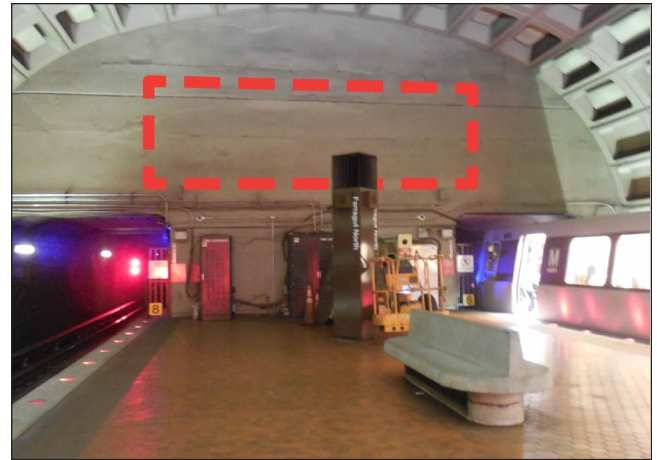
Farragut North Station, southern end of platform, location of pedestrian tunnel connection
