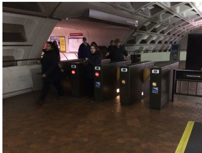
Adding two additional faregates to the Center Mezzanine is part of the station improvements proposed for Farragut North Station
