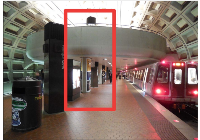
Farragut North Station, Center Mezzanine proposed location of new stair and elevator
