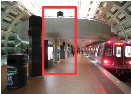
Farragut North Station, Center Mezzanine proposed location of new stair and elevator
