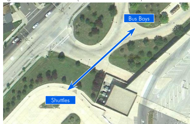
Figure 5: Pedestrian Shortcut (Southern Avenue Station)
