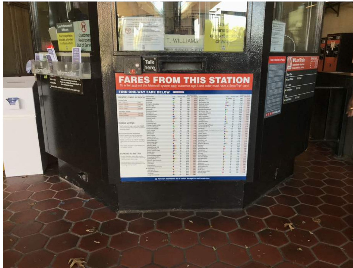
The booth at Huntington Station has many layers of signs added over time. To the degree possible, information should be consolidated while limiting the overall number of signs.
