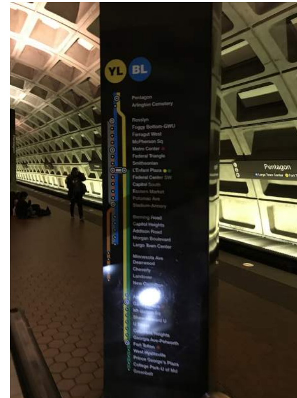
A pylon sign is dimly lit and obscured by glare and shadows from the escalator at Pentagon Station.
