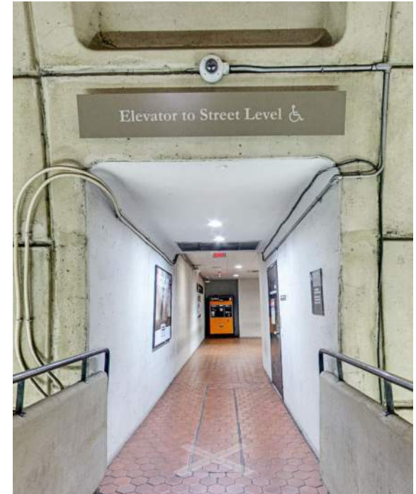
Corridor within signage pointing to elevator at Gallery Pl-Chinatown station.
