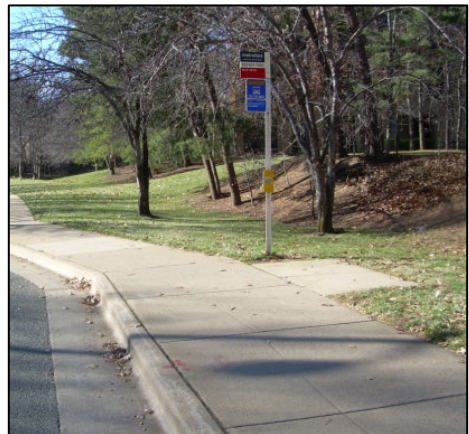
Landing pad on the backside of the sidewalk.
