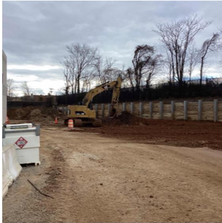
Phase 1 CSX retaining wall, lagging complete
