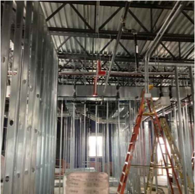
L2 framing and rough-in
