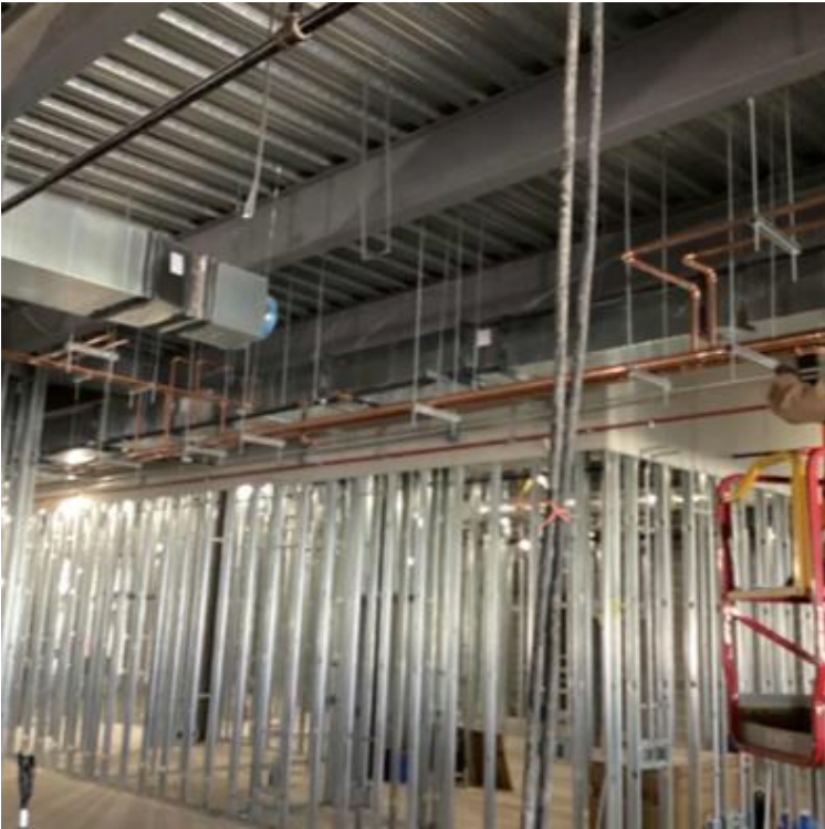
Mezz framing, top of wall drywall installed, rough-in ongoing
