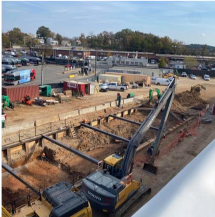
RWH 2-8 Excavation (3rd Lift)
