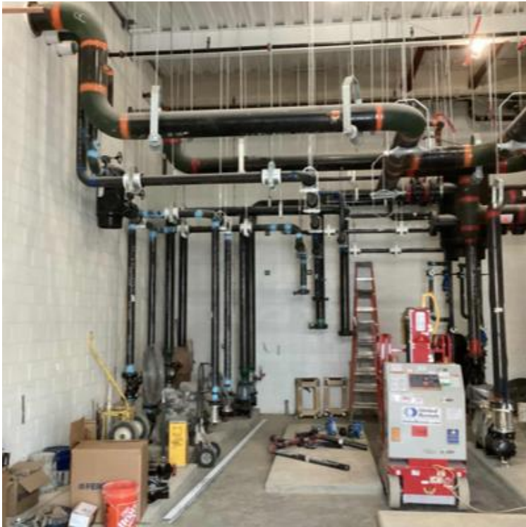
Boiler room rough-in
