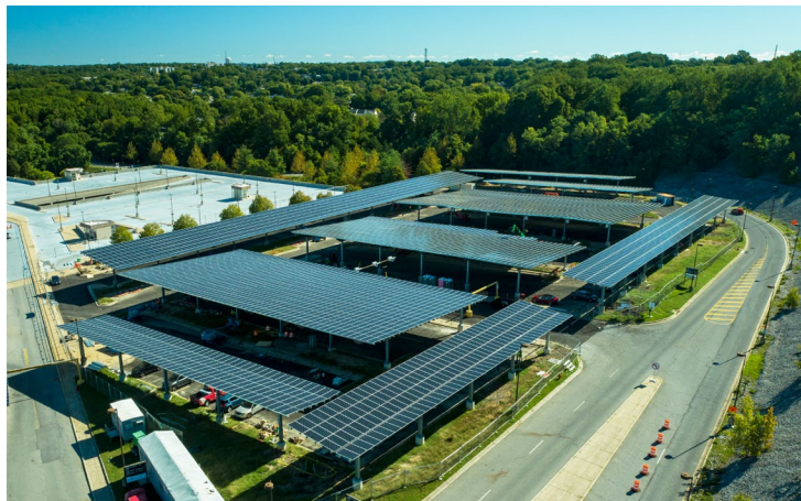
Pictured: Solar carport installation at Southern Ave Metrorail Station
