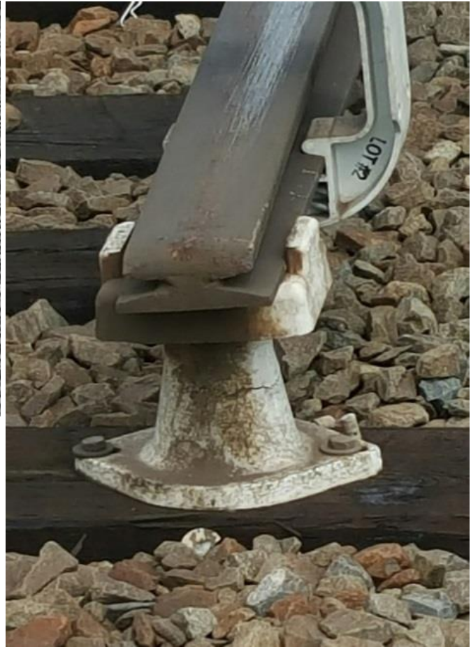
Third rail end with cracked insulator – possibly load imbalance due to curve.
