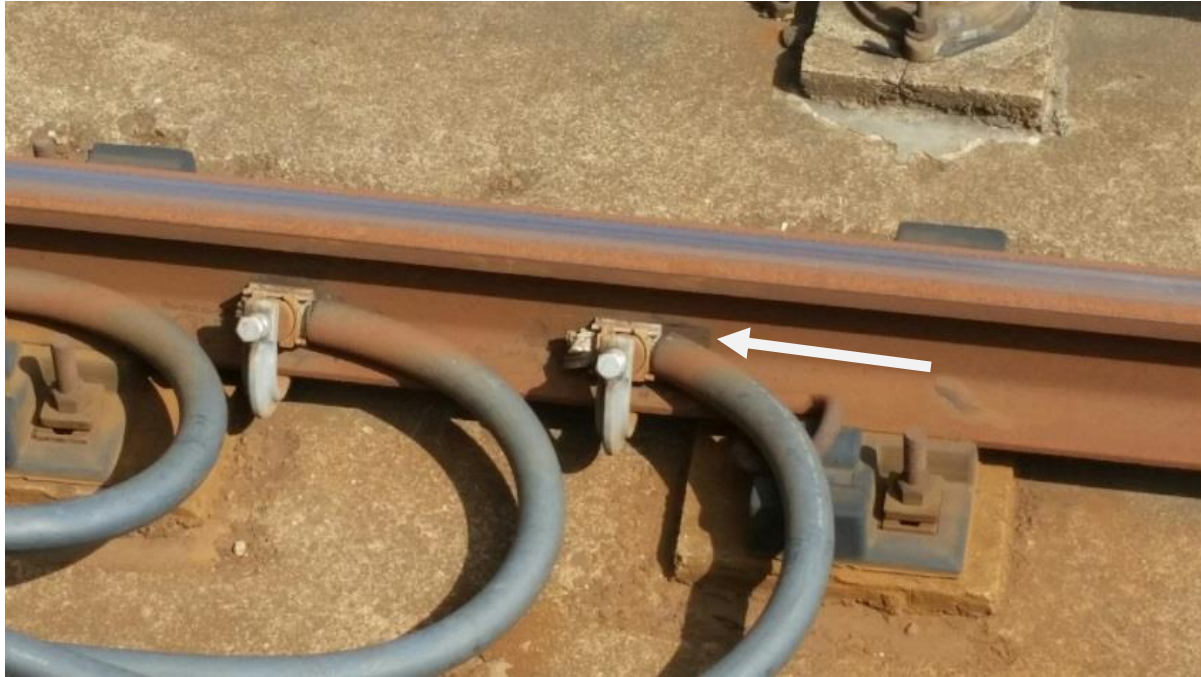
Signal cable clamped to rail, appears to have been in place for extended period of time. One clamp shows movement on rail.
