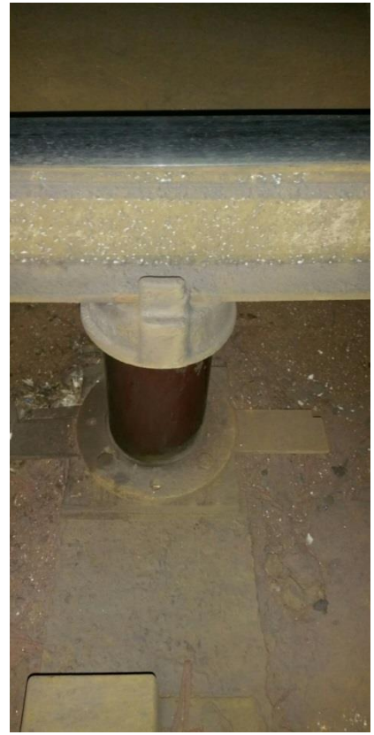
Insulator cleaned and dried
