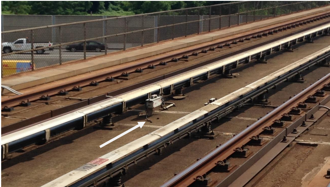
The third rail connection to the heater control panel is off the rail.
