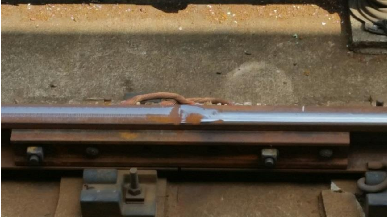
Running Rail Joint "C" bond, appears to be in good condition.
