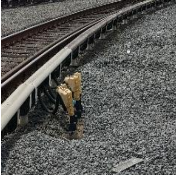
Yard curve with cover board and boots showing wear/age possibly UV issue.
