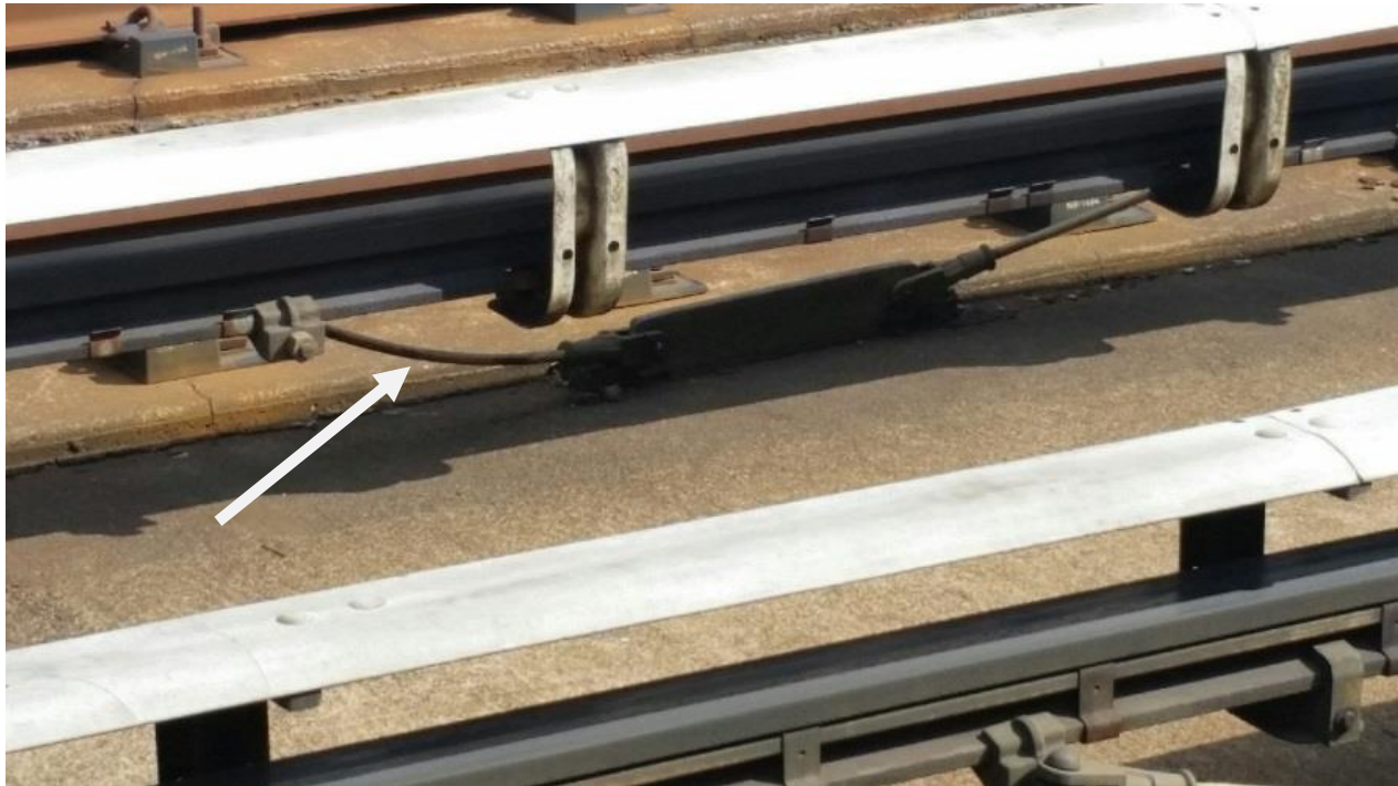
Contact rail anchor improper installation, anchor is bowing due to improper placement of connection on third rail.
