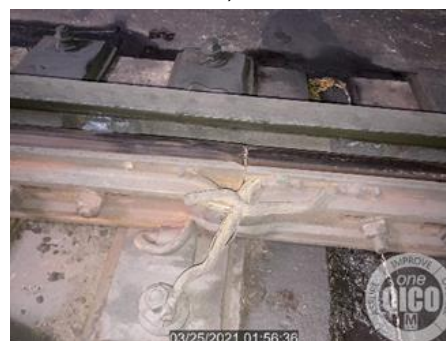
Figure 10: Debris on track bed and rail corrosion
