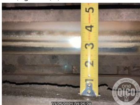
Figure 9: Flangeway gap measurement Over Tolerance
