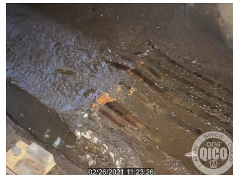
Figure 6: Debris Covering Track Drain Grate
