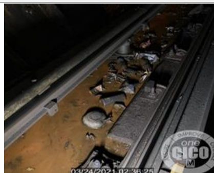
Figure 8: Debris on Track Bed and Rail Corrosion
