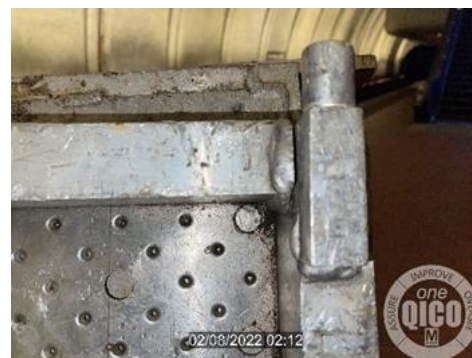
Figure 10: Rail cart with broken weld
