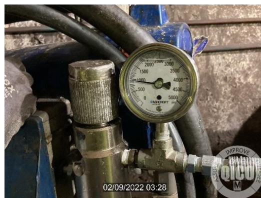
Figure 4: Pressure gauge showing psi while pumping grout into wall
