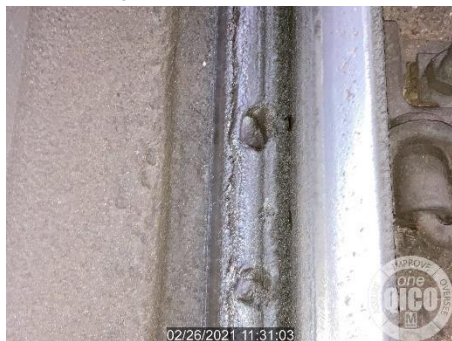
Figure 5: Excess Lubrication Build Up
