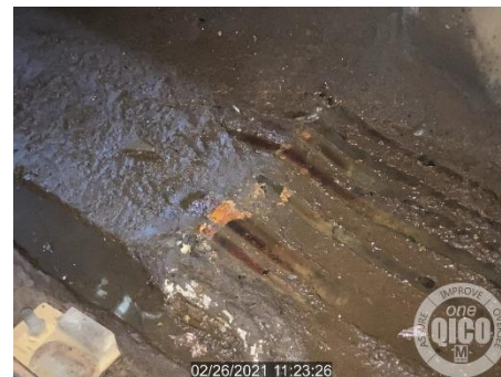
Figure 6: Debris Covering Track Drain Grate
