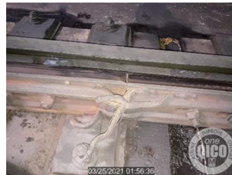
Figure 10: Debris on track bed and rail corrosion
