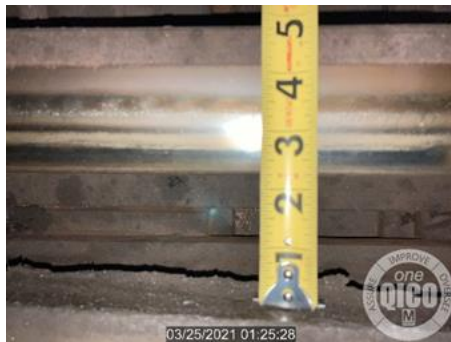
Figure 9: Flangeway gap measurement Over Tolerance
