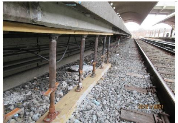
Figure 5: STIN evidence of temporary structures support reinforcement (photo courtesy of STIN)
