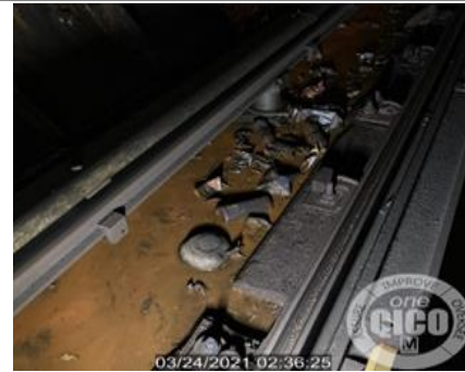
Figure 8: Debris on Track Bed and Rail Corrosion
