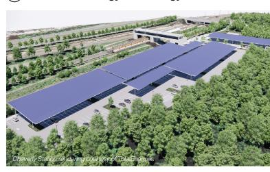
Solar carports are overhead canopies built of steel that support solar panels which collect sunlight, a renewable energy source, that is converted to electricity. The electricity will be sent to the utility company and finally delivered to local homes and businesses.
