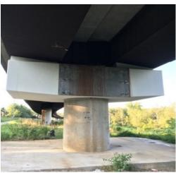
"Hammer heads" help extend the life of the aerial structures by strengthening the connections between the column and beams, improving the load capacity and preventing additional deterioration due to train vibrations.
