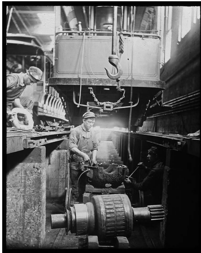
(6) University of Cincinnati Motor Repair Work Traction Company Foote, Elmer L., Photographer
