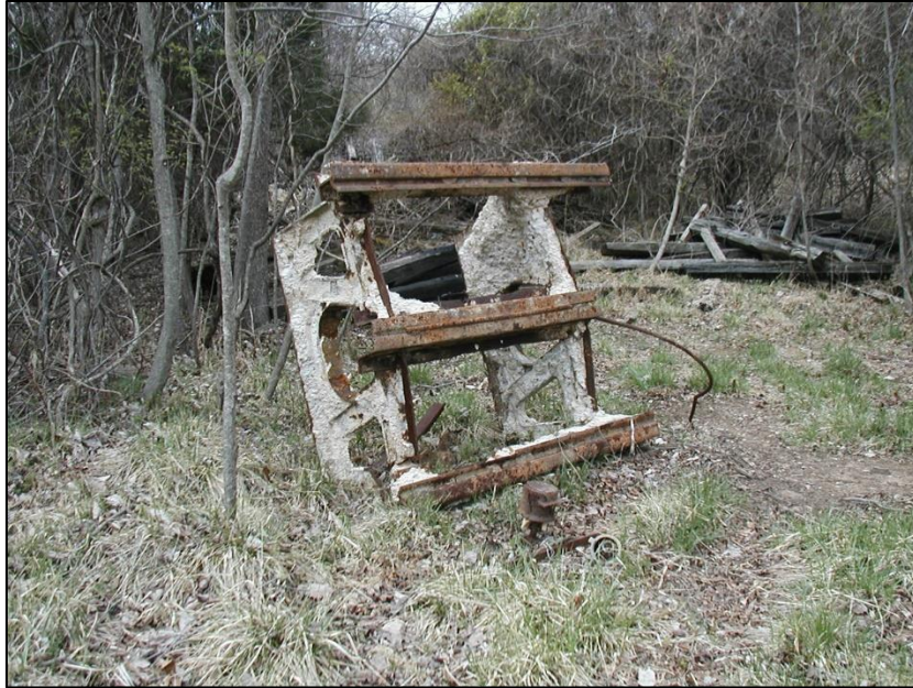
(9) Abandoned Excavated Yoke and Tracks https://www.dctrolley.org/history
