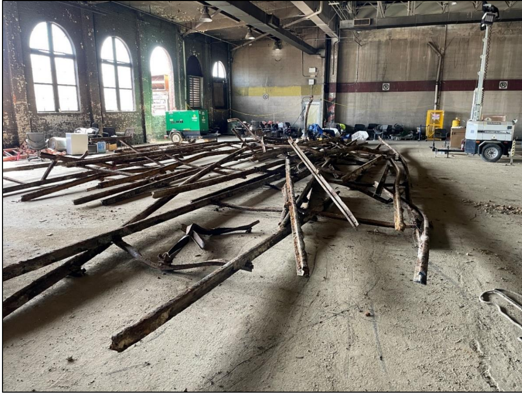
(7) Northern Bus Garage interior, embedded tracks removed from floor. May 2023
