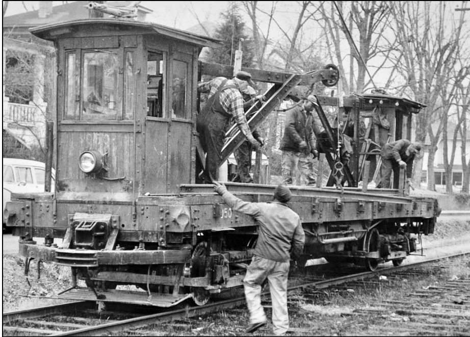
(7) Removing DC Streetcar Tracks, 1960
