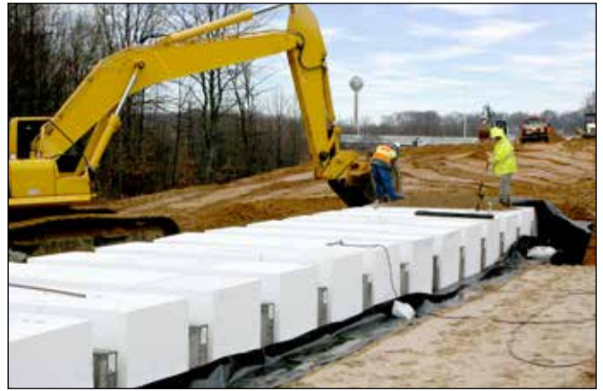
EPS Geofoam Protection
