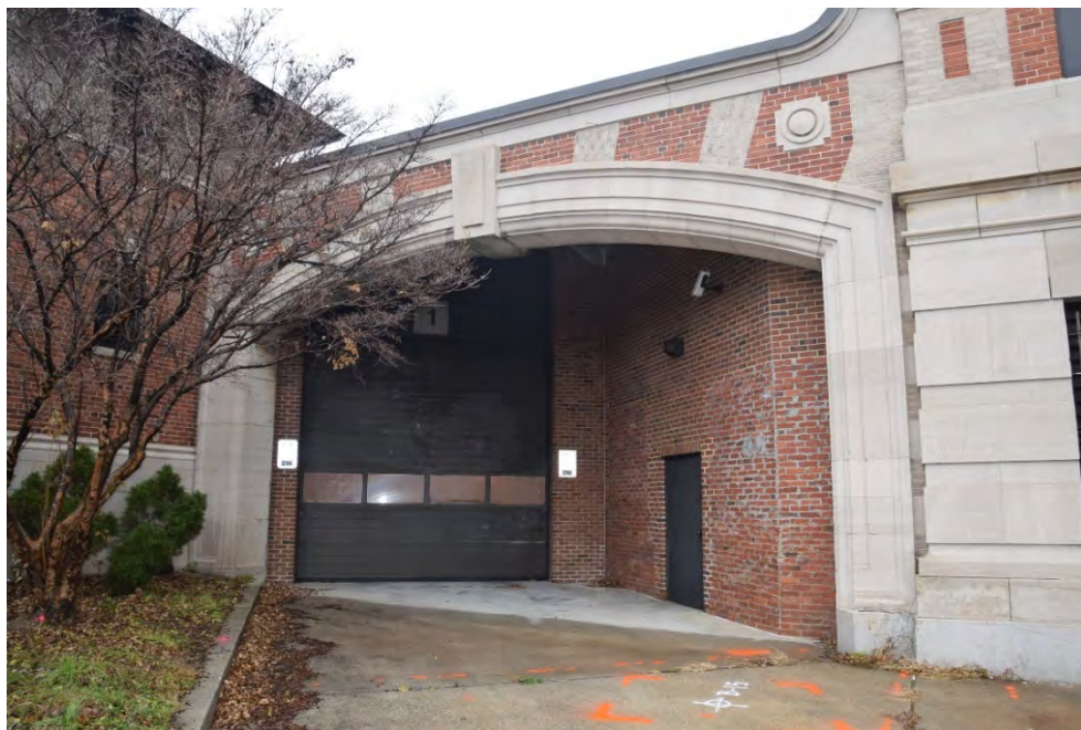
Figure 8. Angled brick wall on right constructed sometime after 1914 and prior to 1978. The wall created an additional interior room and enclosed the north elevation of the tower at that level. The other angled wall with the overhanging door was added after 1978 (BBB)
