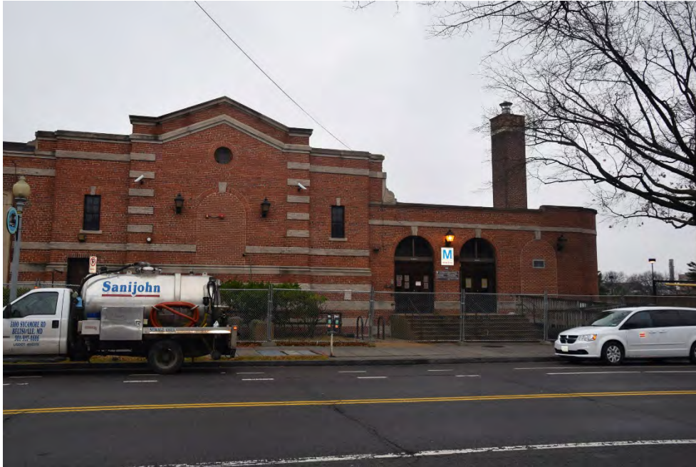
Figure 13. Two doorways to the right of the pedimented bay are non- historic. Left window opening changed to door prior to 1974 and right window changed to a door during the 1987-1992 renovation (BBB)
