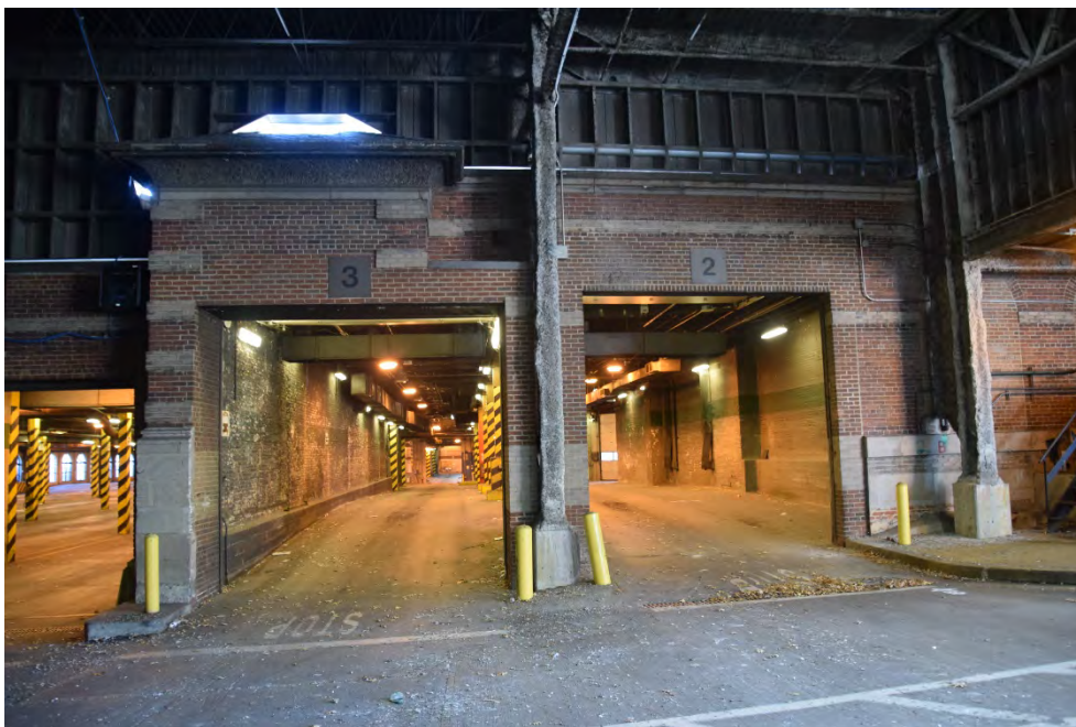
Figure 14. A truncated roof shelters the original north elevation and Decatur Street. Large openings for buses were punched in the wall during the 1987-1992 renovation (BBB)
