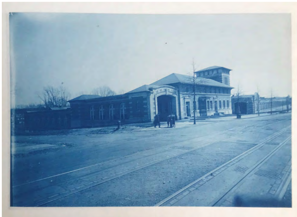
Figure 3. 1914 exterior photograph of the northwest corner of the streetcar barn showing the administrative offices, tower, and two of the three original streetcar openings. The north elevation features arched window openings and hipped roof pavilions at the center and western corner of the elevation (DC History Center)
