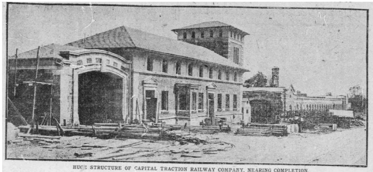
Figure 1. 1906 photograph of the car barn and administrative offices during construction (Washington Times)
