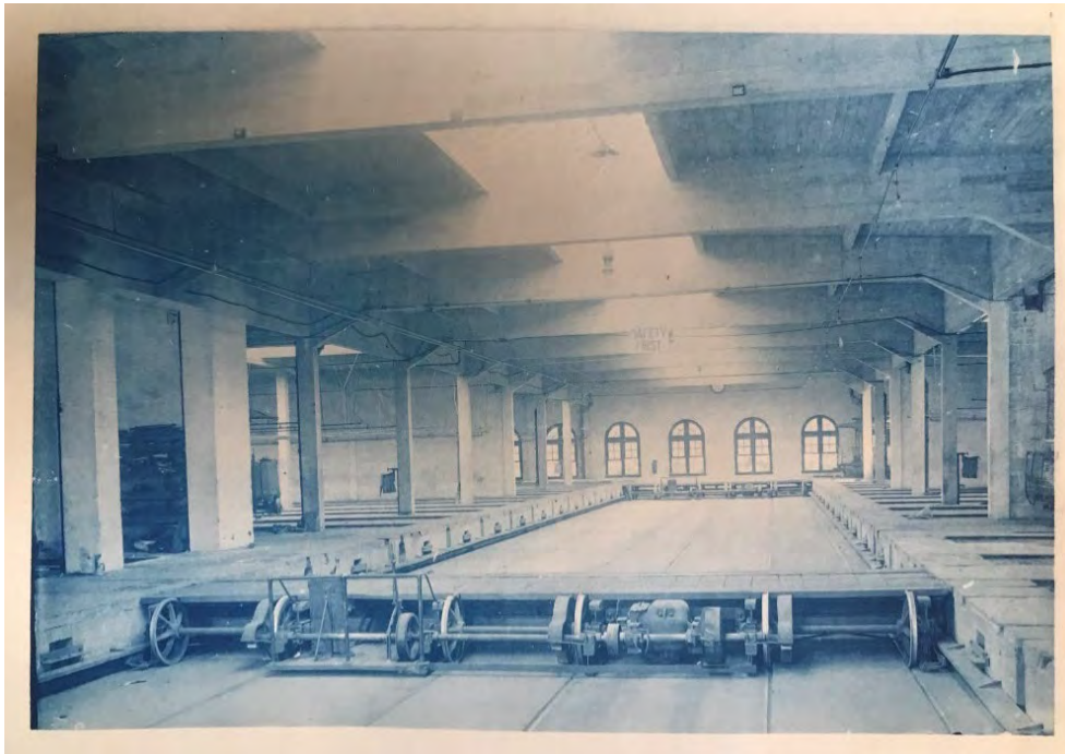
Figure 4. 1914 interior photograph of the Decatur Streetcar Barn showing the transfer table in the foreground and the skylight above (DC History Center)
