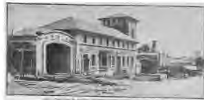
"Large Structure of Capital Traction Railway Company, Nearing Completion". 1906 Washington Times
