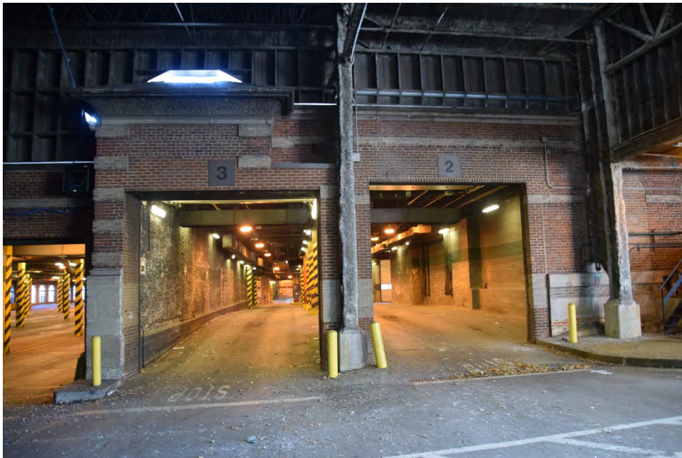
Figure 14. A truncated roof shelters the original north elevation and Decatur Street. Large bus openings punched in wall during the 1987-1992 renovation (BBB)
