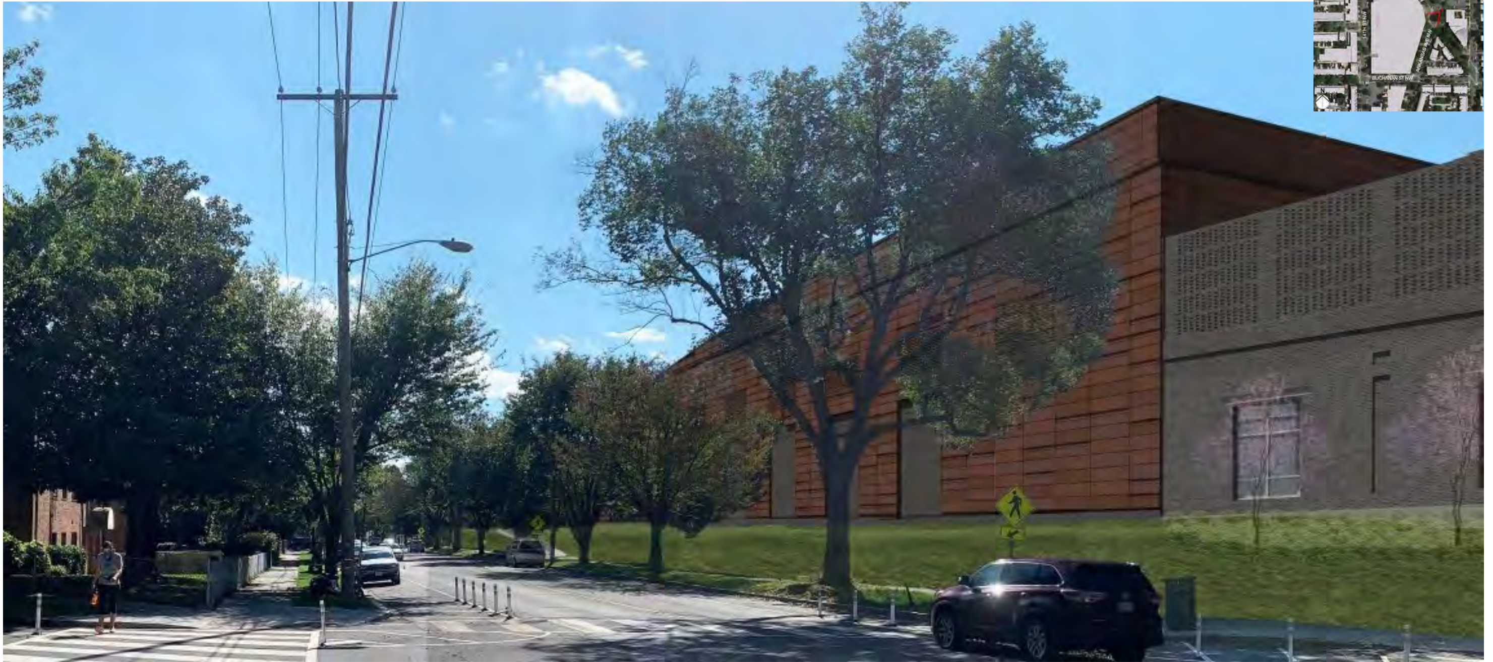
VIEW LOOKING SOUTHWEST ALONG ARKANSAS
