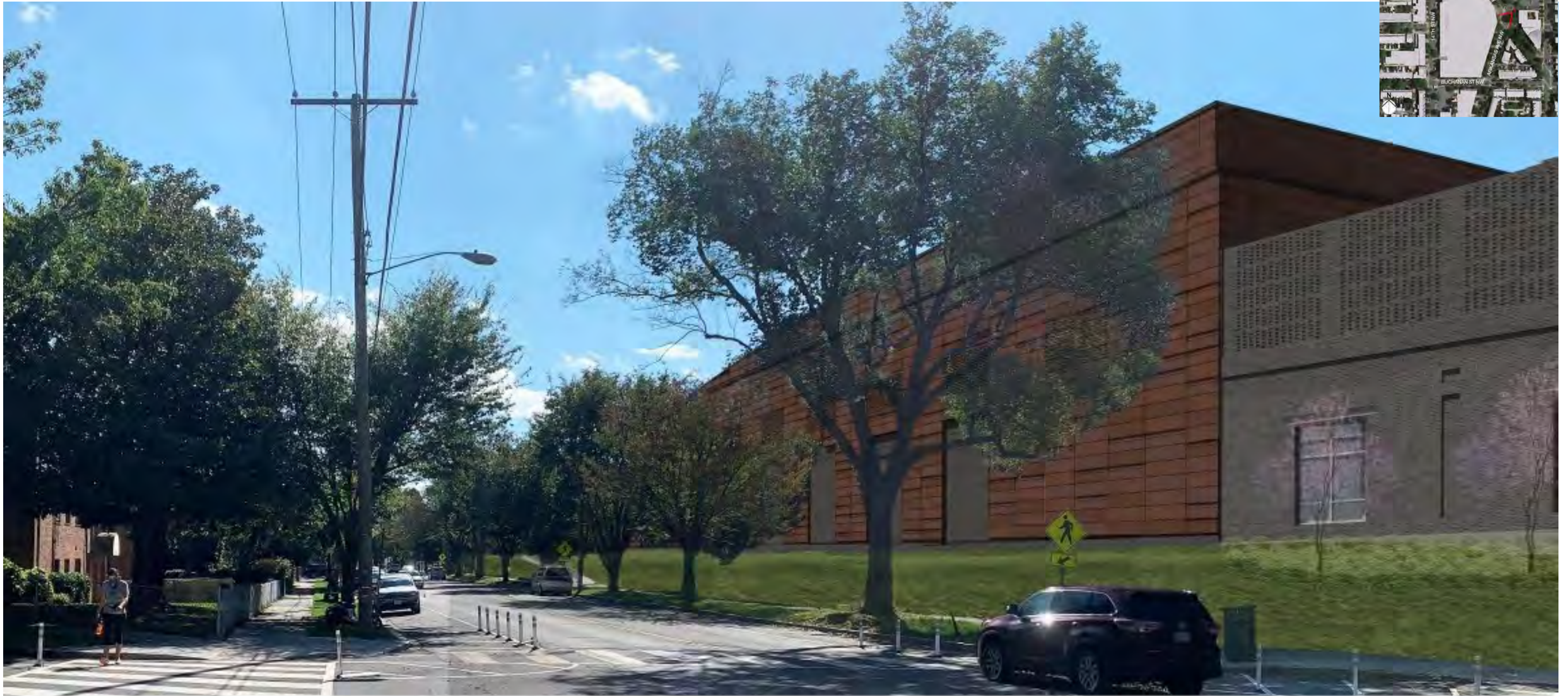
VIEW LOOKING SOUTHWEST ALONG ARKANSAS
