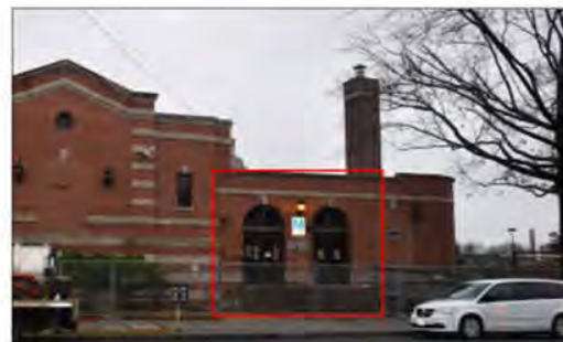
1980s Doors to be Restored to Windows
