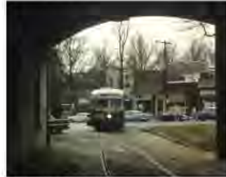
3963 View of Trolley from Car Barn
