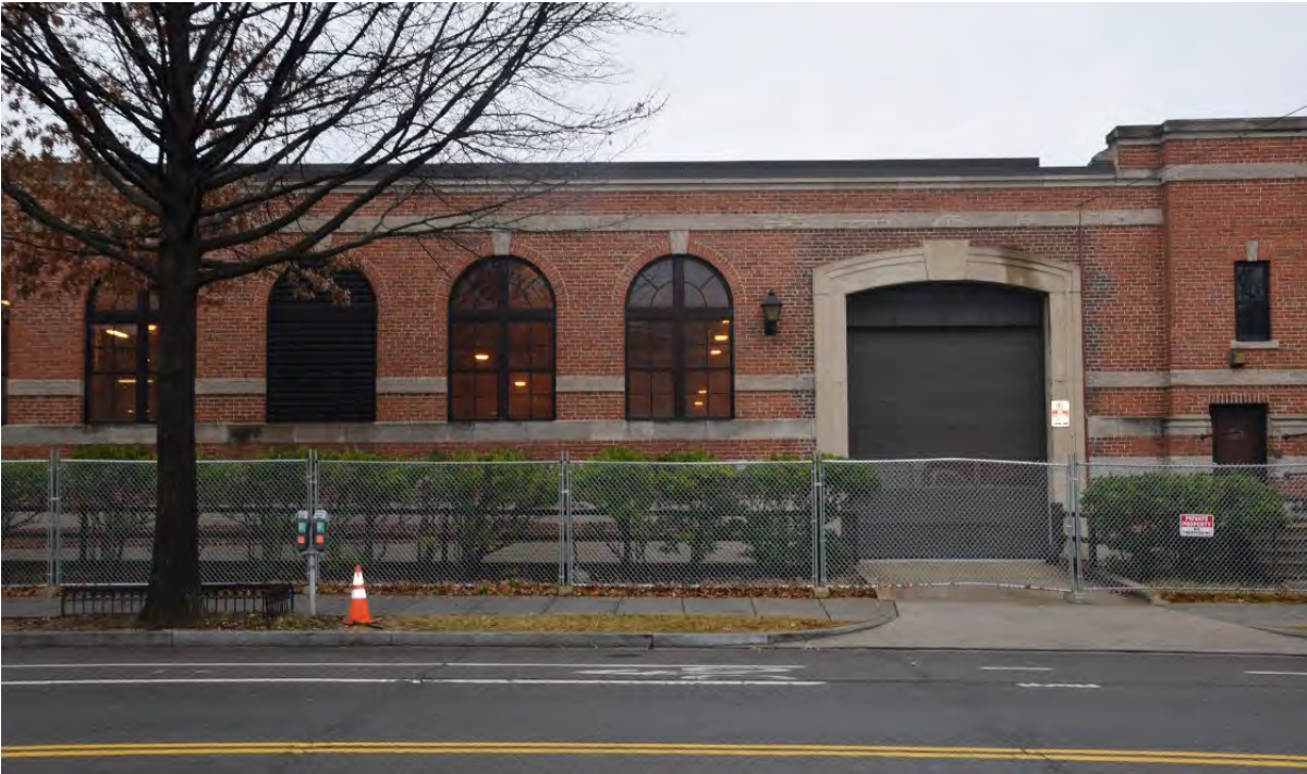
Figure 12. Bus entry at the southern end of the west façade added during the 1987-1992 renovation (BBB)
