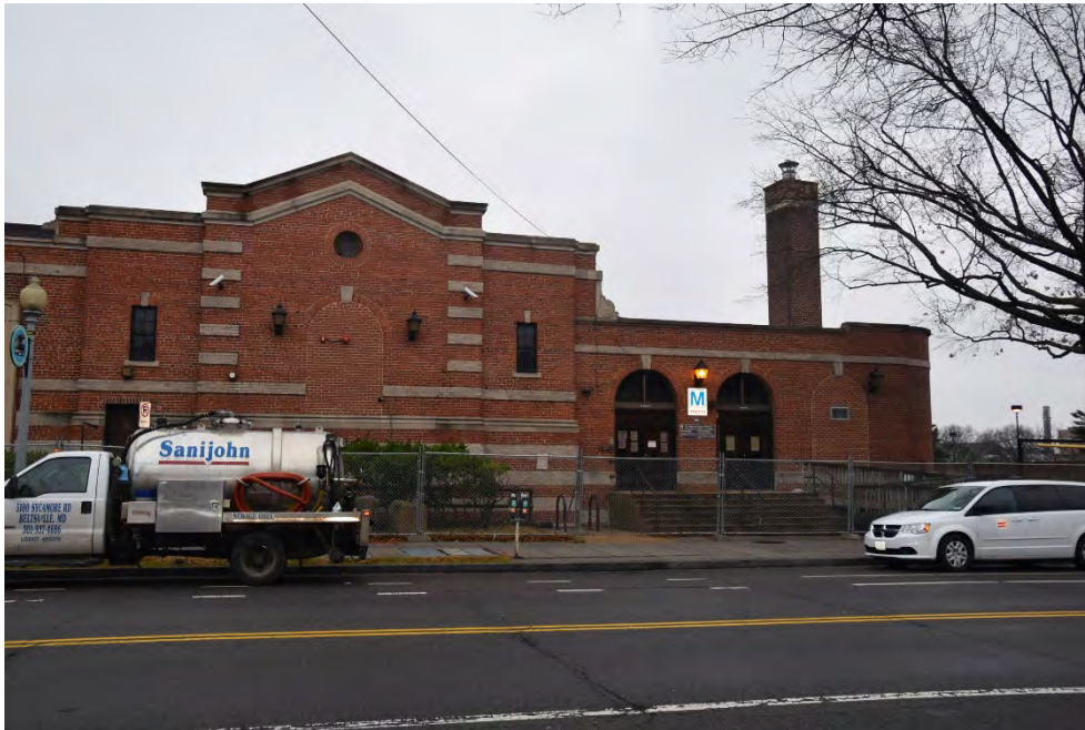
Figure 13. The two doorways to the right of the pedimented bay are not historic. The one on the left was changed from a window opening to a door prior to 1974 while the one on the right was changed during the 1987-1992 renovation (BBB)
