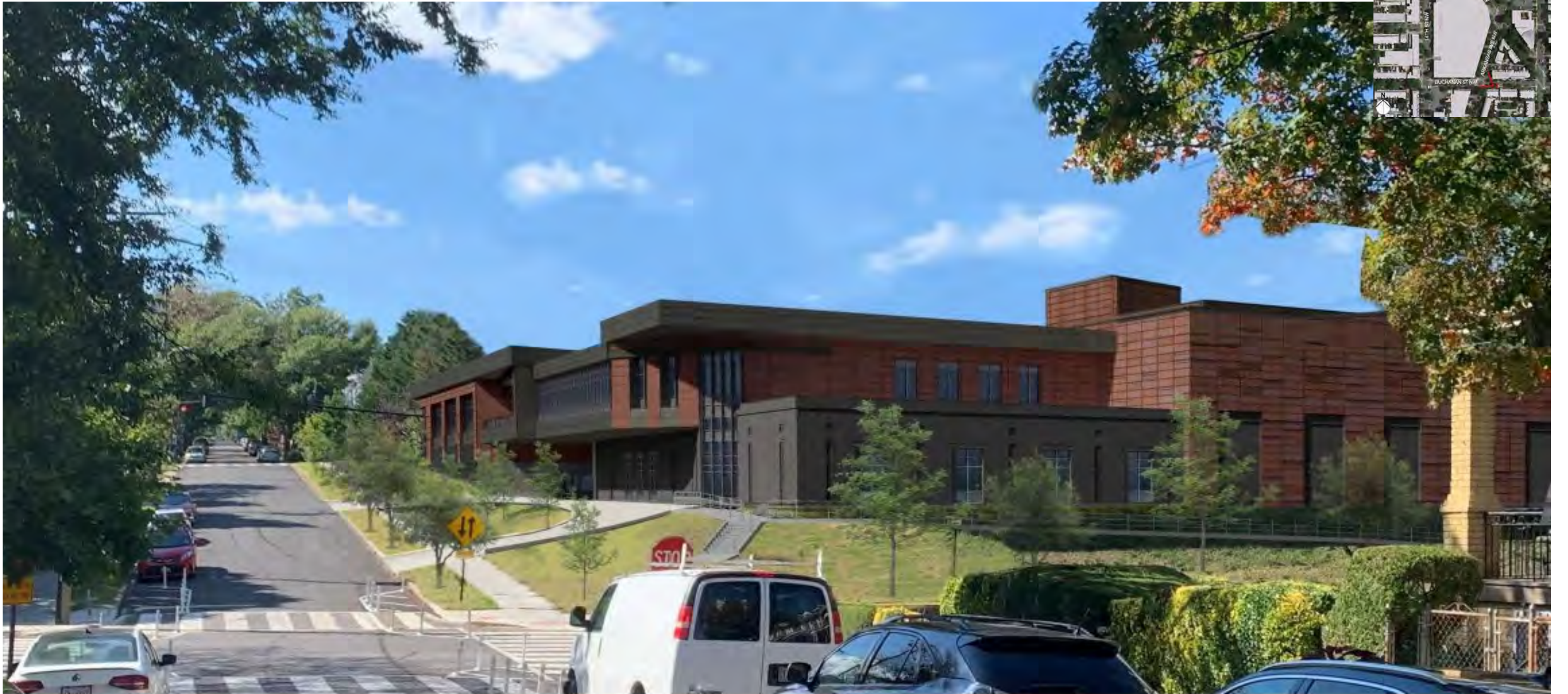
VIEW LOOKING WEST ALONG BUCHANAN AT SOUTHEAST CORNER
