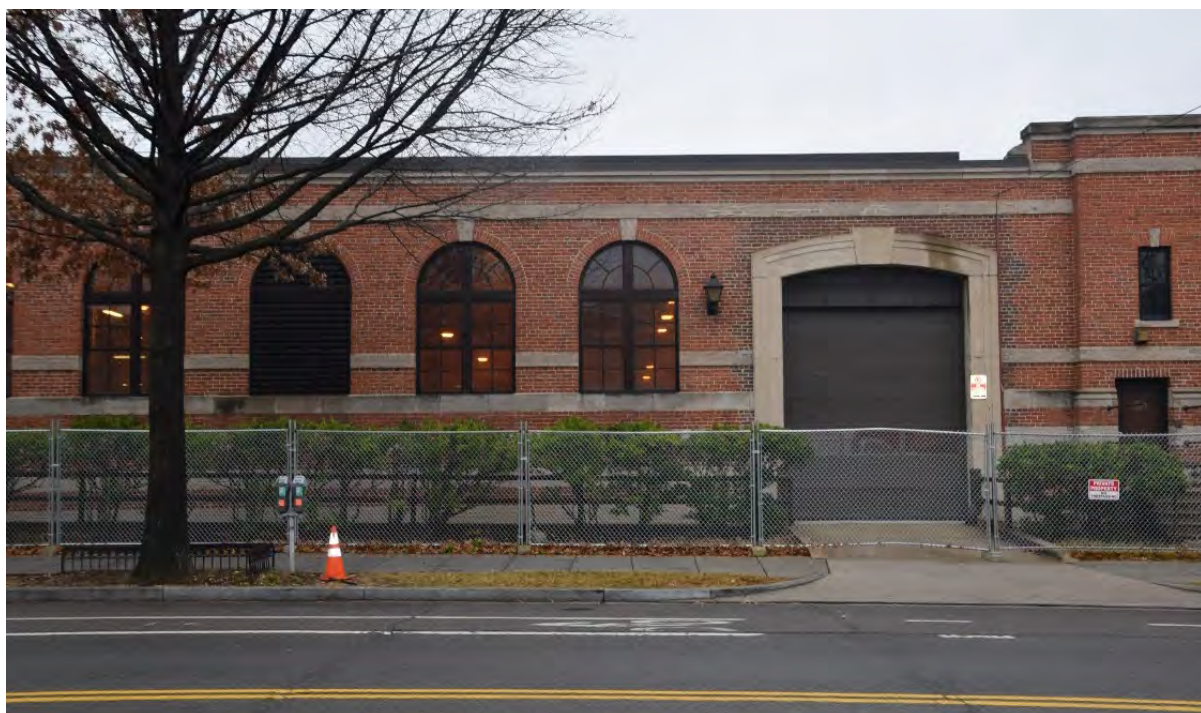
Figure 12. Bus entry at the southern end of the west façade was added during the 1987-1992 renovation (BBB)
