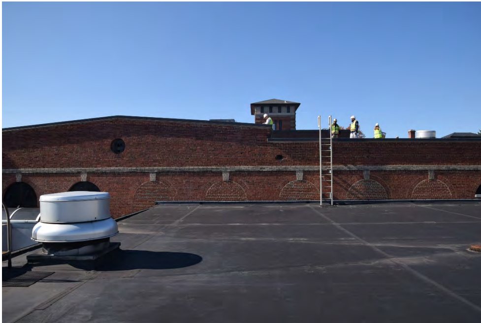
Figure 15. Roof of the 1987 addition abuts the original east elevation. Several of the arched windows have been infilled with brick (BBB)
