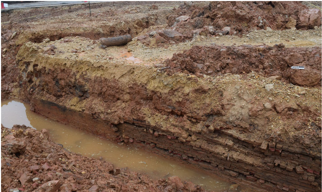
Figure 1. Brick and Mortar Foundation, Southwest Corner.
