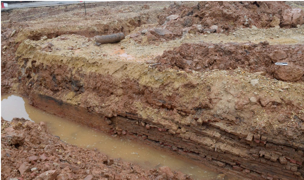
Figure 1. Brick and Mortar Foundation, Southwest Corner.
