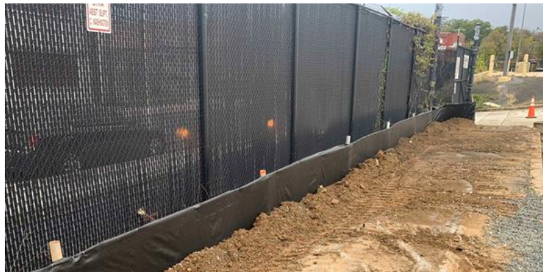
Installation of erosion and sediment controls (super silt fence)
