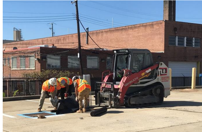
Installation of erosion and sediment controls
