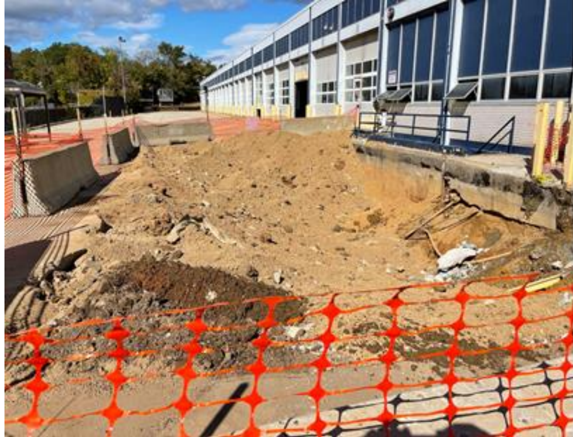
Underground storage tank removal (after)
