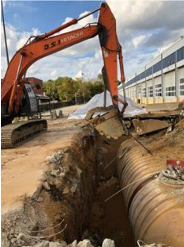
Underground storage tank removal (before)
