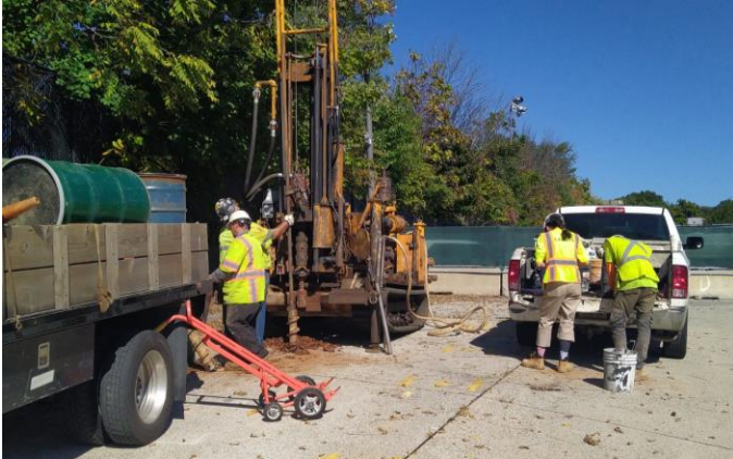
Geotechnical core drilling
