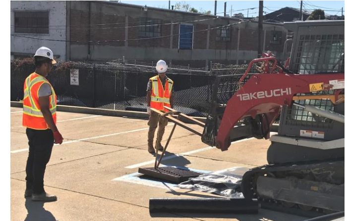
Installation of erosion and sediment controls
