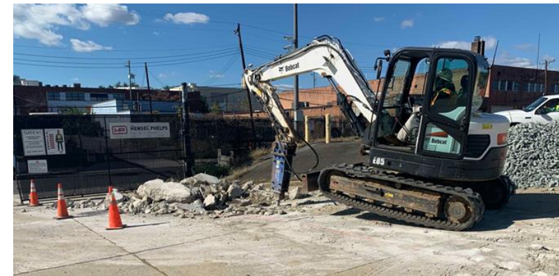
Installation of erosion and sediment controls (stabilized construction entrance)
