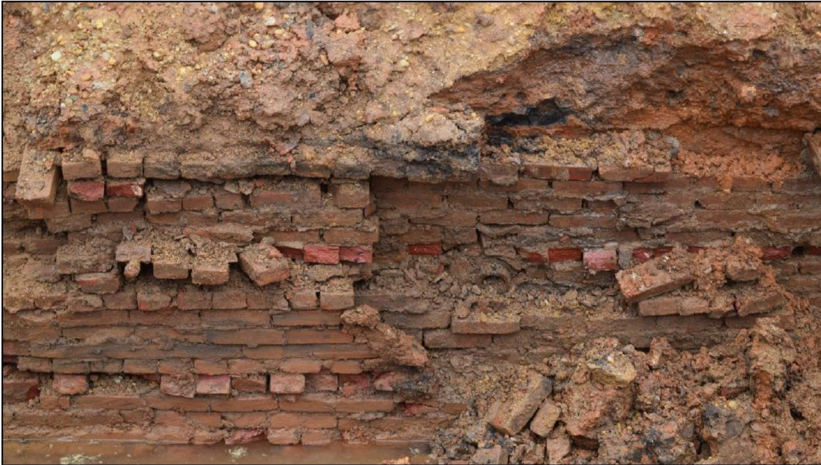
Figure 3. In Situ Brick and Mortar Foundation.
