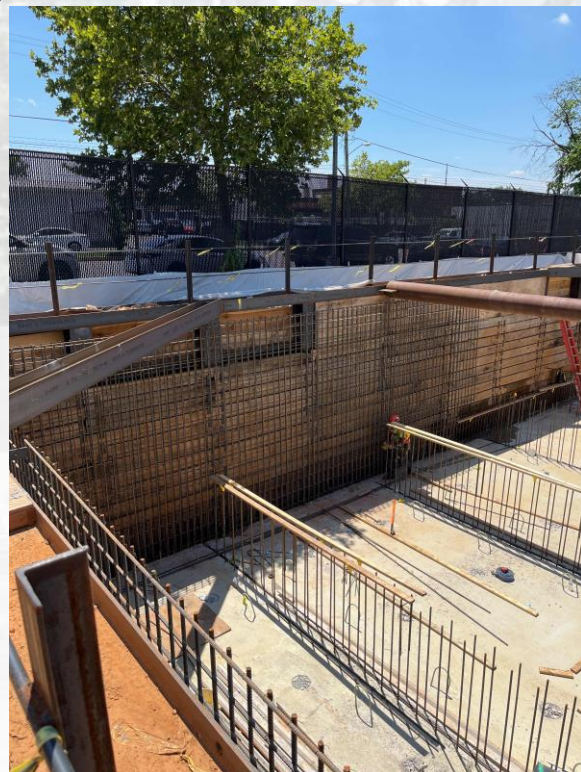
Installed perimeter wall reinforcing steel
