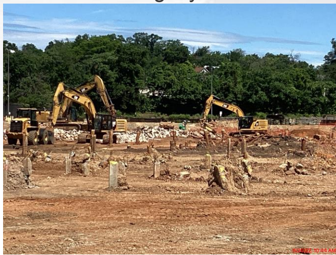
Removal of Micro Piles & Legacy Foundations
