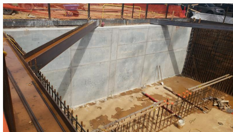
Placed wall section #1
