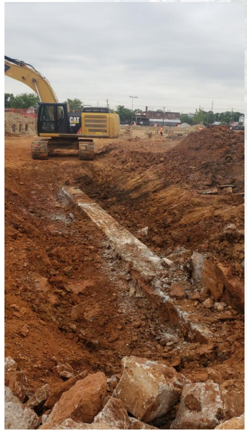
Removal of Legacy Foundation
