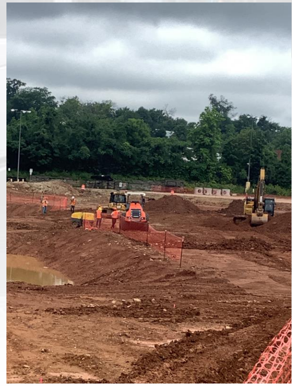
Rough grading / sealing building pad unimpacted areas
