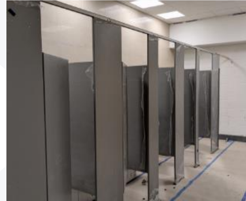
Restroom Partition Install
