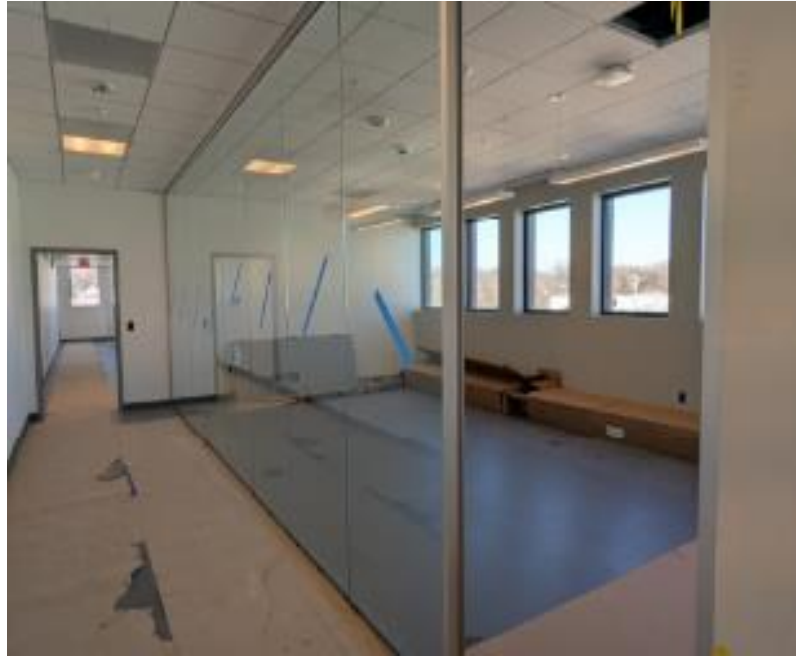
Demountable Partition Install
