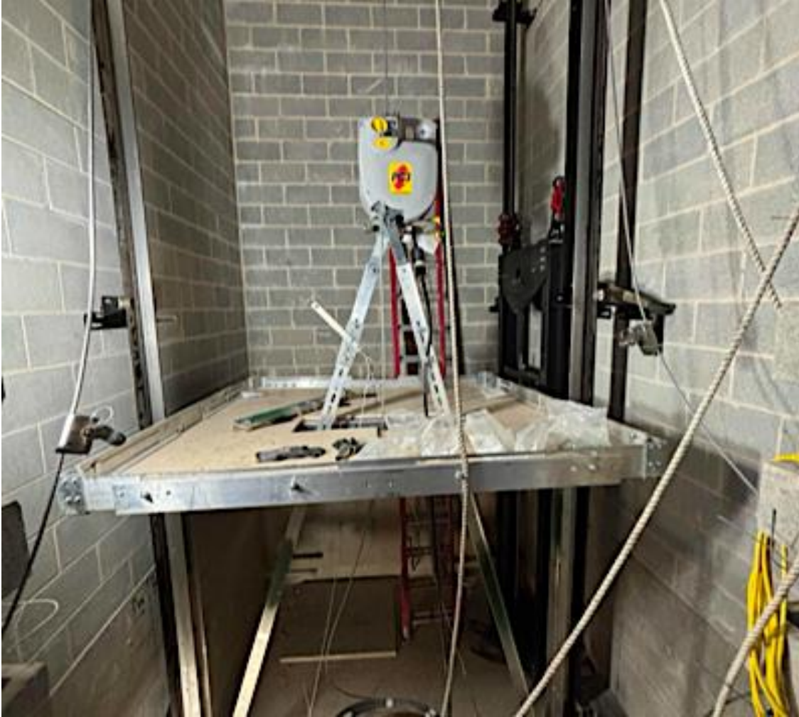
Elevator Platform Install
