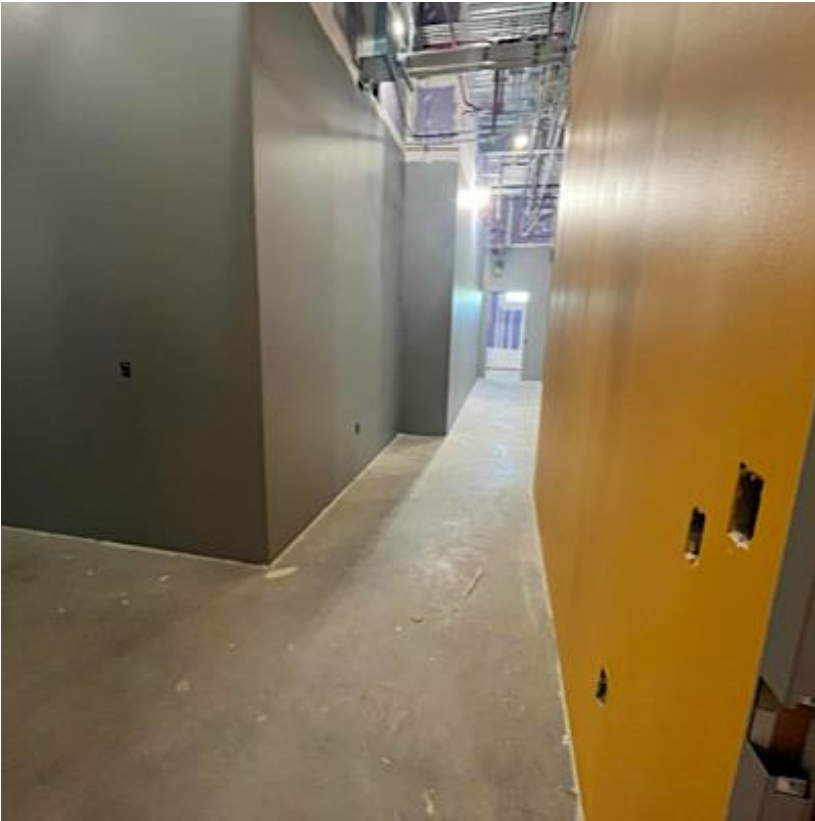
Interior 1st Coat Mezz. Level
