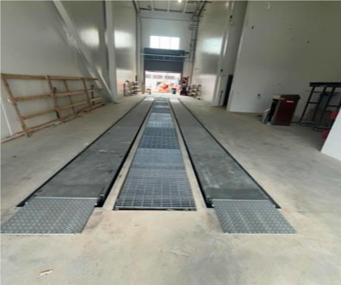
Vehicle Lift Chasis Wash Area
