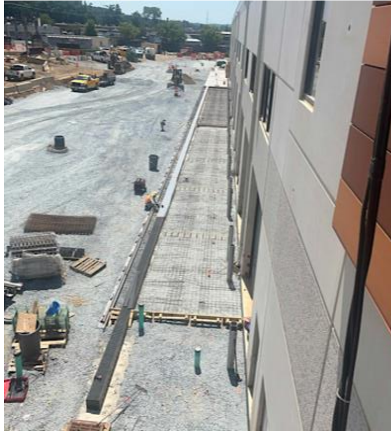
Reinforcement & formwork concrete paving
