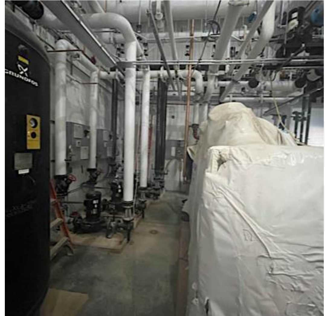
Boiler Room Completed Insulation
