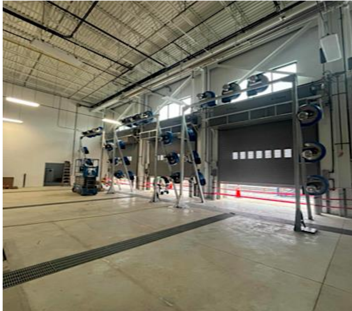
Vehicle Wash Dryer Install
