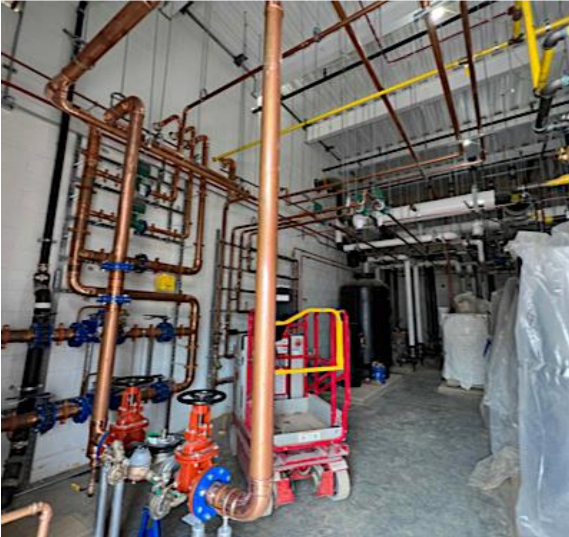
Boiler Room Hot Water Loops
