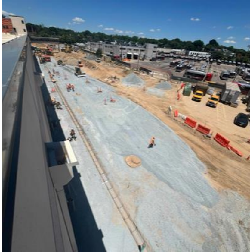
Site prep for concrete paving
