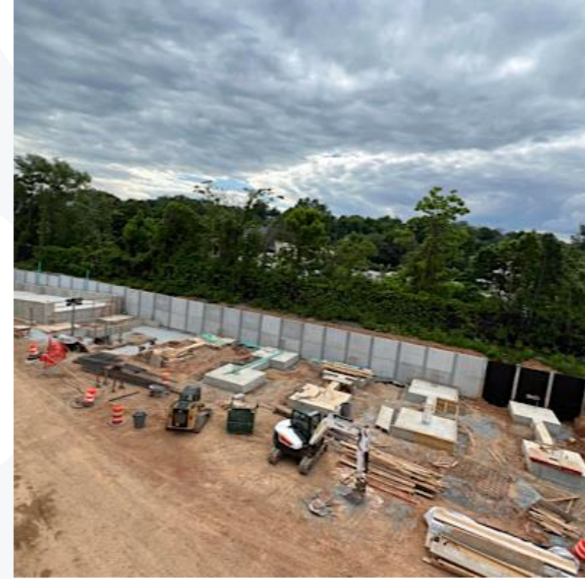
Ramp Foundations In-Progress
