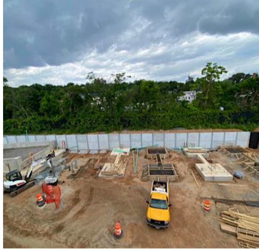
Ramp Foundations In-Progress
