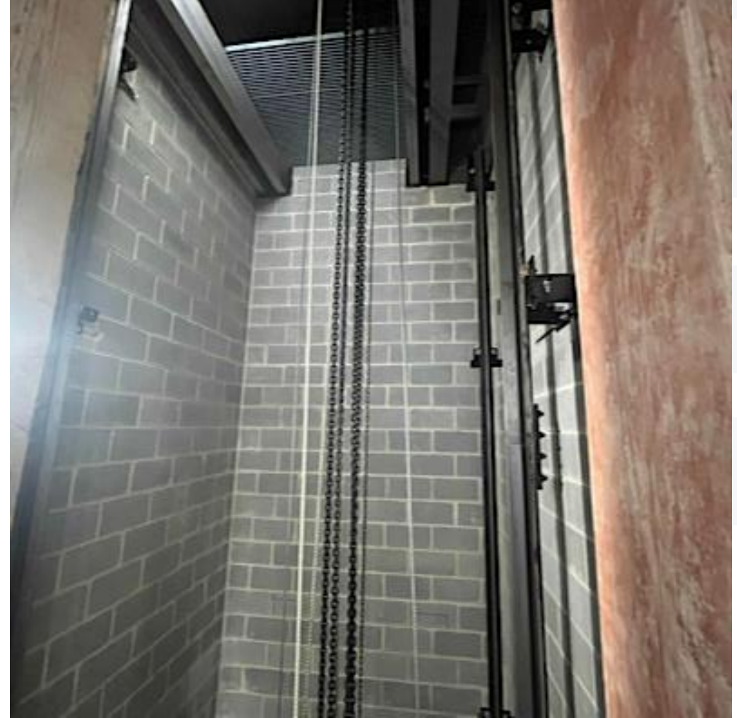
Elevator Rails and Temp Hoisting Cables
