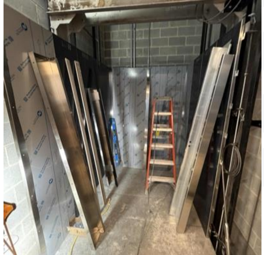
Elevator Cab Build Out 10/7/24
