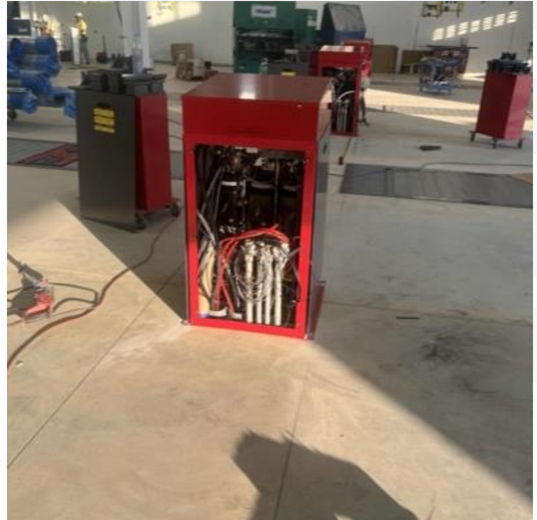
Vehicle Lift Control Panel Set & Tie-In In Progress 10/7/24
