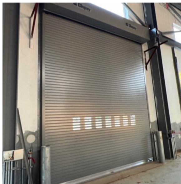
Overhead door install started
