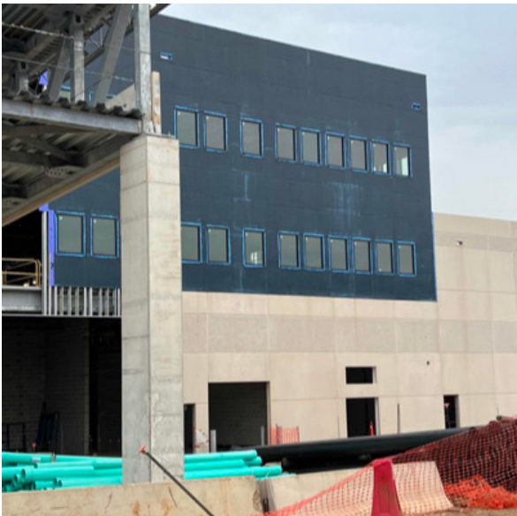
Glazing install ongoing
