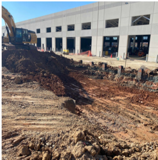
Start of Excavation
