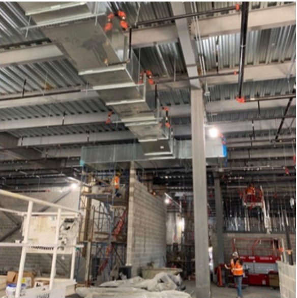
Overhead mechanical / electrical & plumbing ongoing
