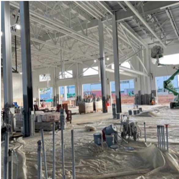
First coat of paint
