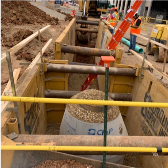
Site utilities started
