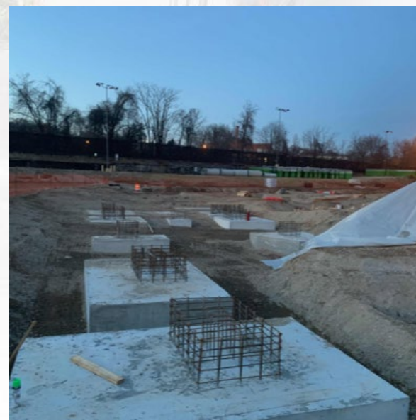
Placed & Stripped Pile Caps
