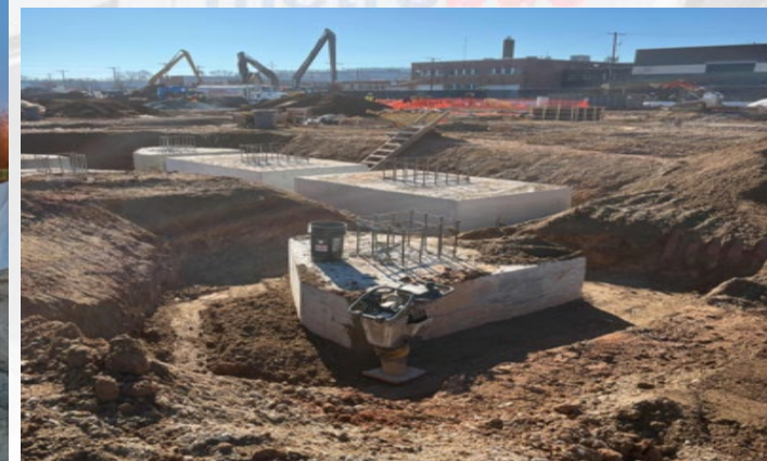
Pile Cap Backfill
