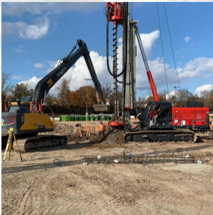
Fixed Mast Auger Rig
