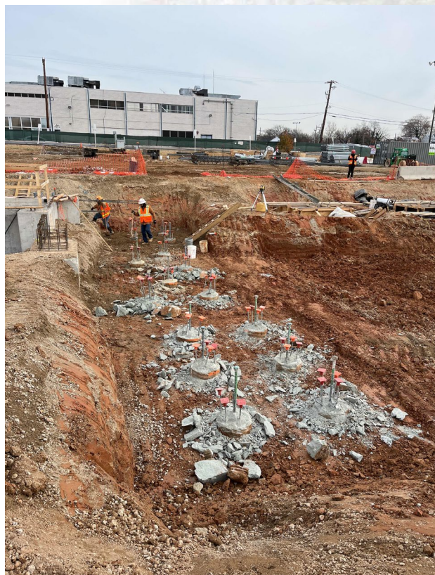
Prep For Pile Caps
