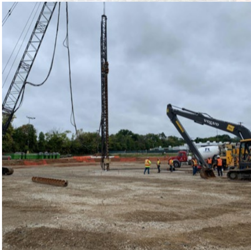
Start of Auger Cast
