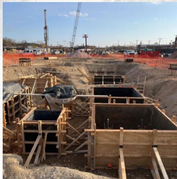
Pile Cap Formwork
