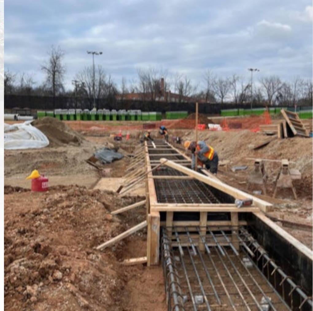
Grade Beam Formwork
