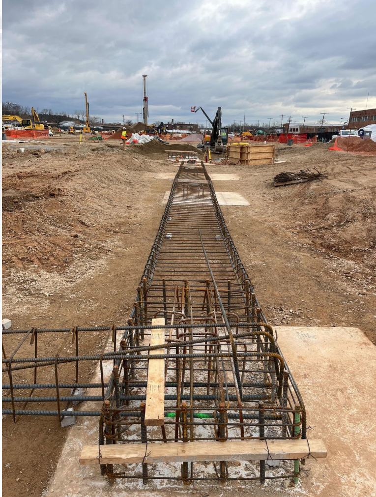
Grade Beam Reinforcing
