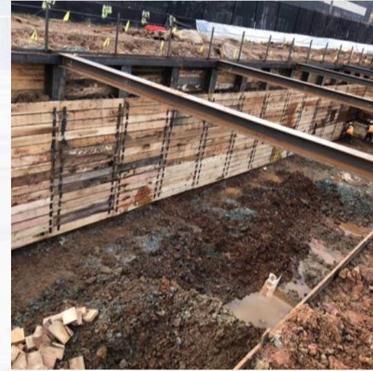
RWH 1-6 Third Cut
