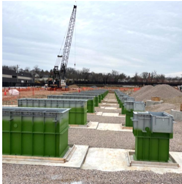
Ready for Grout
