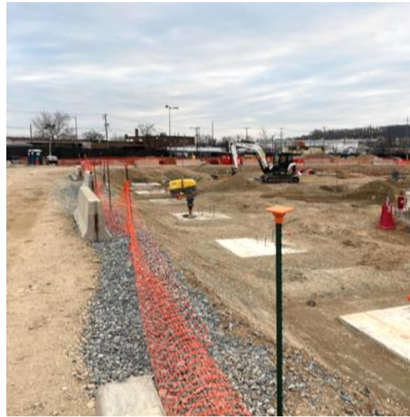
Backfill Around Pile Caps
