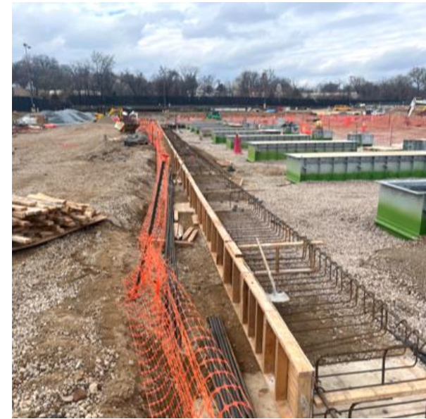
Continuation of Grade Beams
