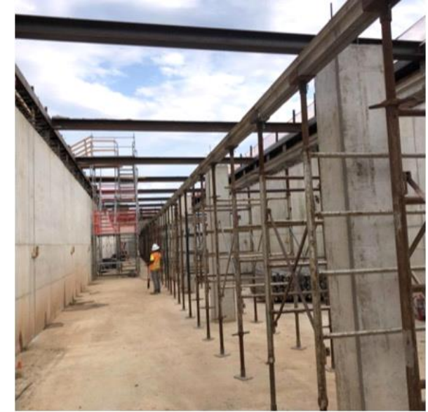
Center Beam Shoring
