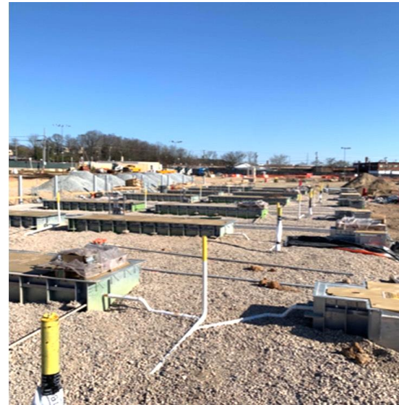
Backfilled & Utility Connections Complete
