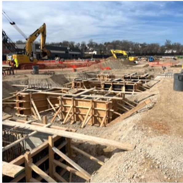
Final Pile Caps
