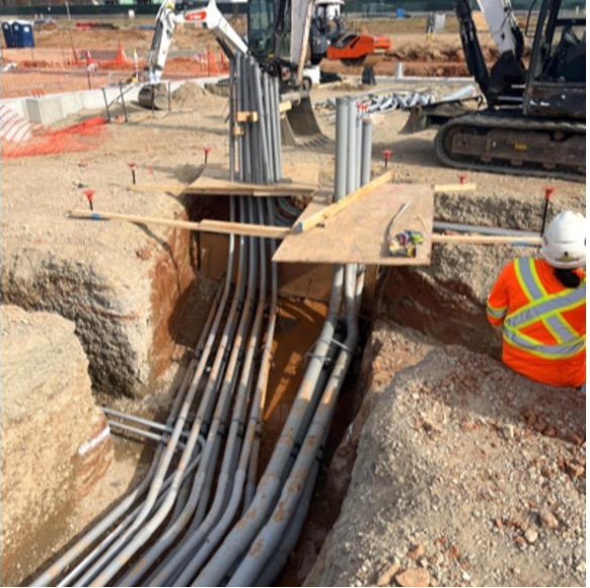
Underground Ductbank
