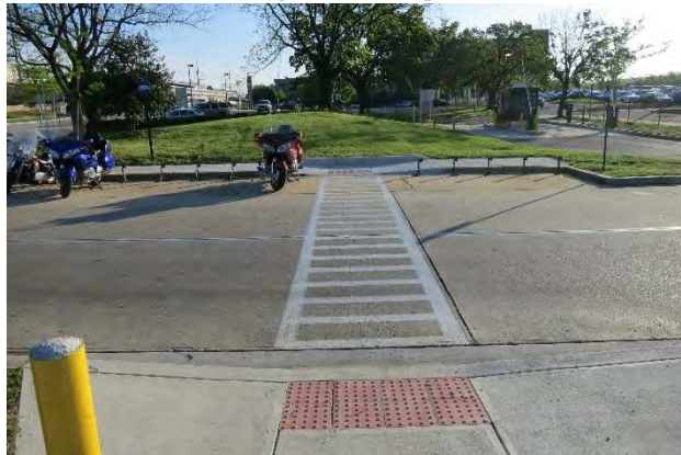
Figure 103: Egress Driveway Crosswalk at Motorcycle Parking Area
