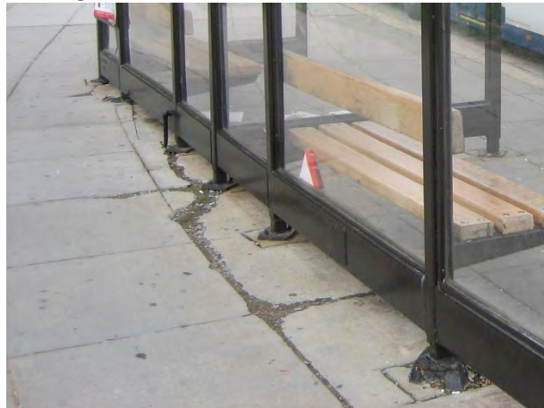
Figure 75: Poor Pad Condition, Shelter A
