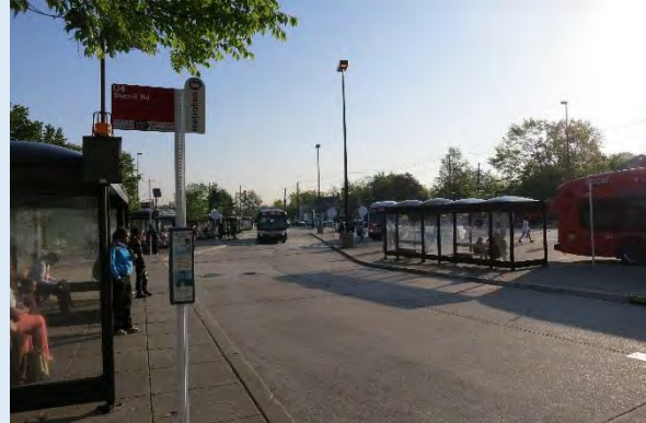
Busway Between Platforms
