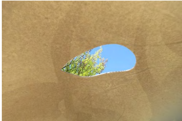
Figure 180: Hole in Dome Top, Shelter G South
