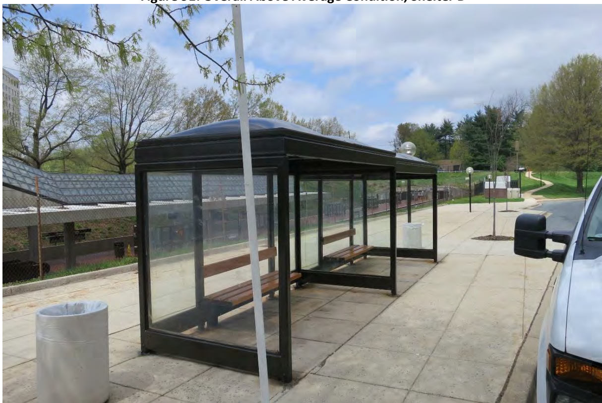
Figure 91: Overall Above Average Condition, Shelter D
