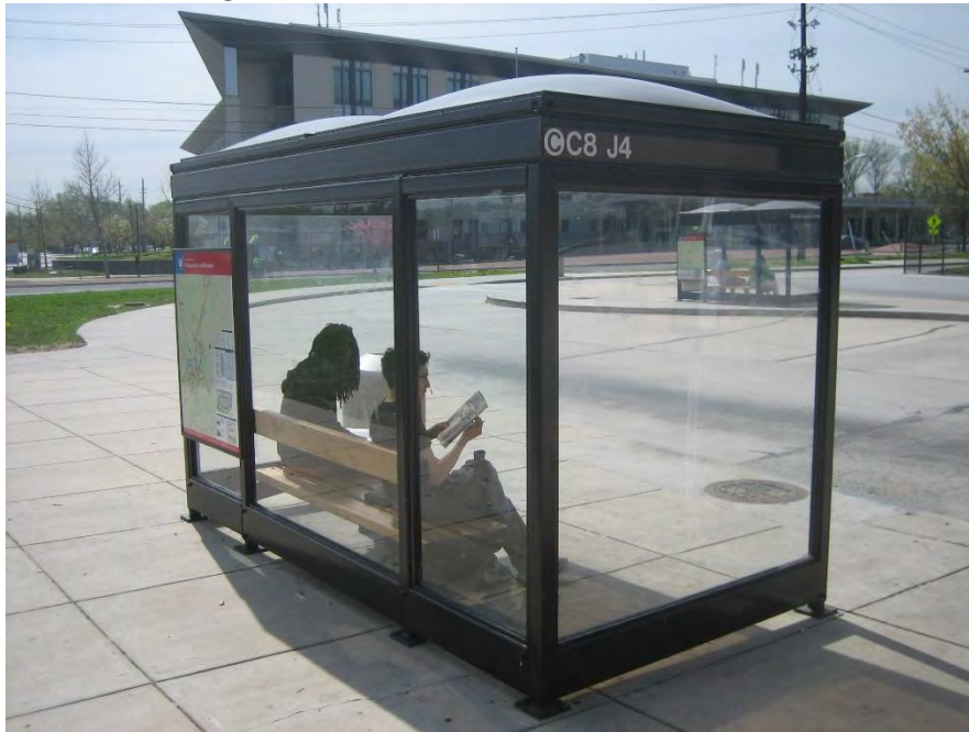
Figure 44: Good Overall Condition, Shelter C
