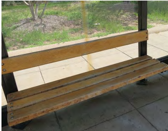
Figure 63: Faded/Scratched Panels, Kiss & Ride Shelter
