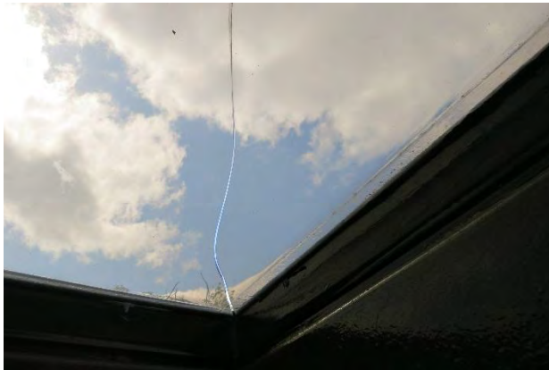
Figure 155: Cracked Dome Top, Shelter C
