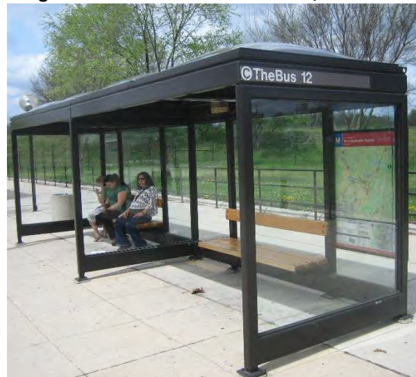
Figure 187: Good Frame Condition, Shelter C
