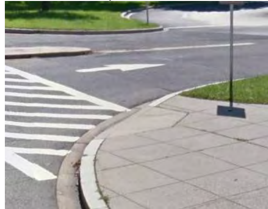
Curb Ramp at Eastern Avenue
