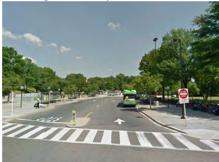
Figure 117: Busway from Cedar Street
