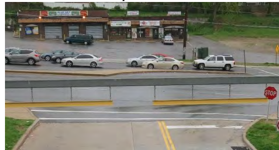
Left-Turn Bay on Central Avenue
