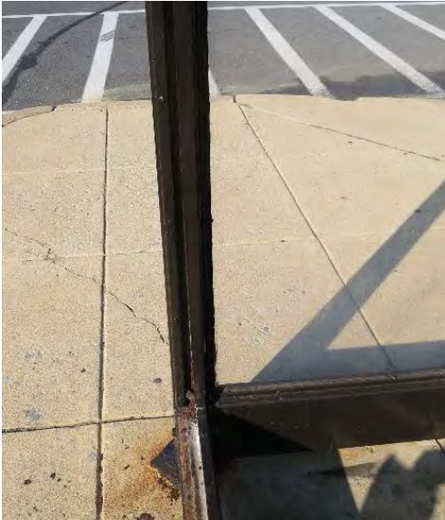
Figure 103: Frame Rust, Shelter D
