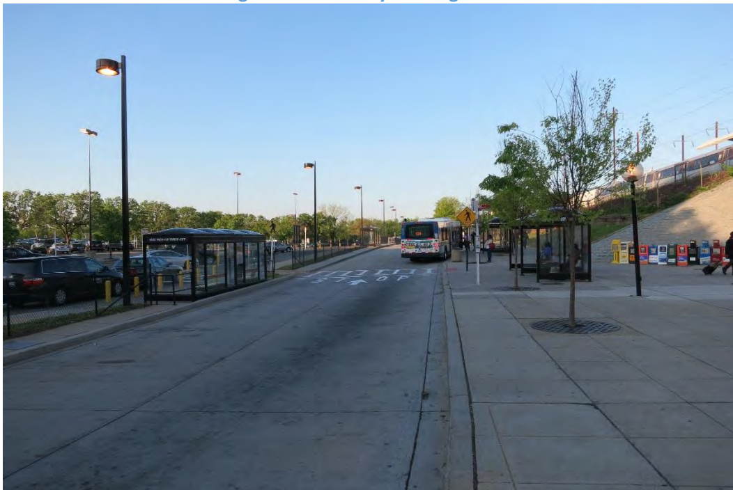
Figure 111: Busway Looking South
