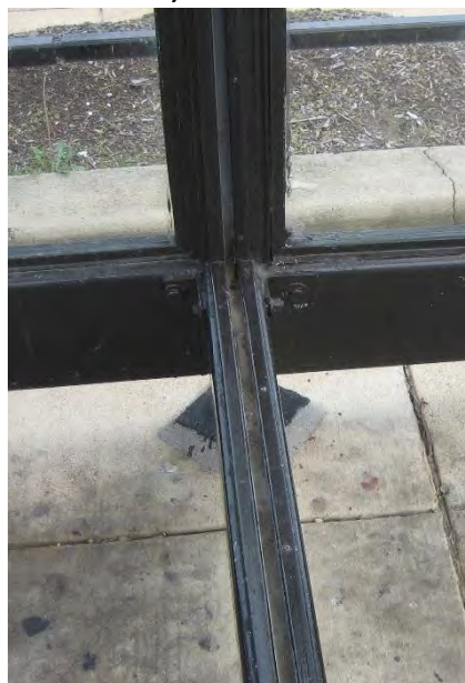
Figure 35: One of Two Missing Panels, East Kiss & Ride
