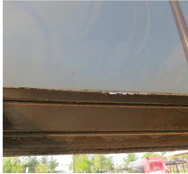
Figure 58: Frame Rust and Separated Dome Top, Kiss & Ride Shelter
