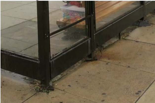
Figure 4: Cracked Pad, Shelter B
