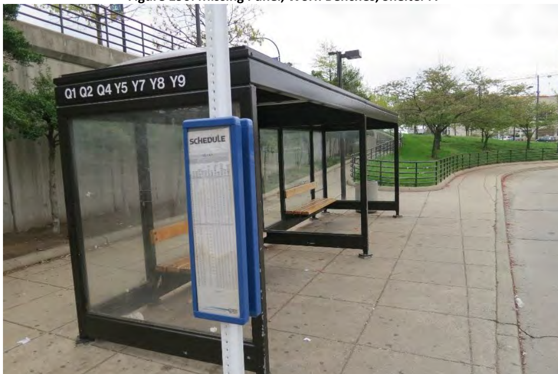
Figure 190: Missing Panel, Worn Benches, Shelter A
