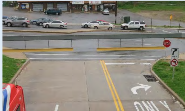
Crosswalk Traversing Central Ave Entrance Driveway
