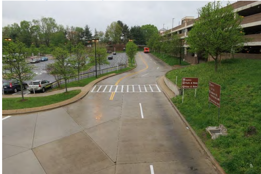
Figure 16: Busway Exit at Central Avenue Driveway
