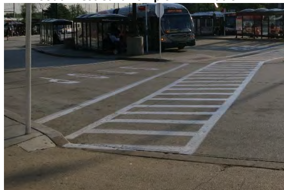
Southwest Curb Ramp on A-H Platform
