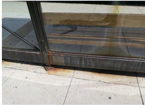
Figure 63: Faded/Scratched Panels, Kiss & Ride Shelter
