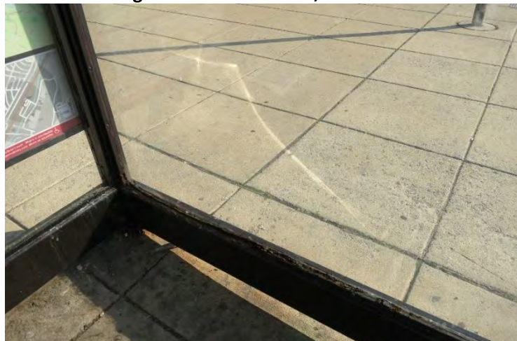
Figure 103: Frame Rust, Shelter D
