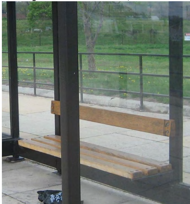
Figure 186: Wear on Bench, Shelter A
