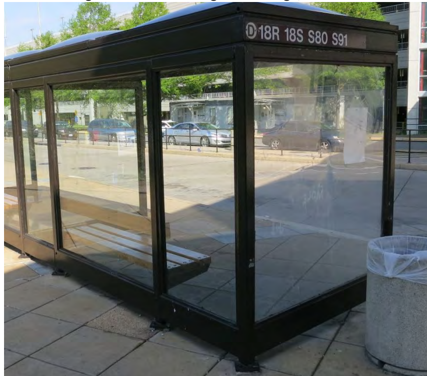
Figure 81: Panel Fading and Damage, Shelter D
