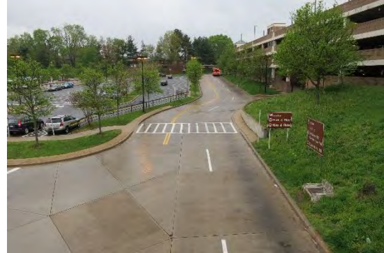
Crosswalk Traversing Central Ave Entrance Driveway
