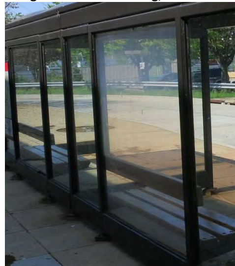
Figure 69: Panel Fading, Shelter D
