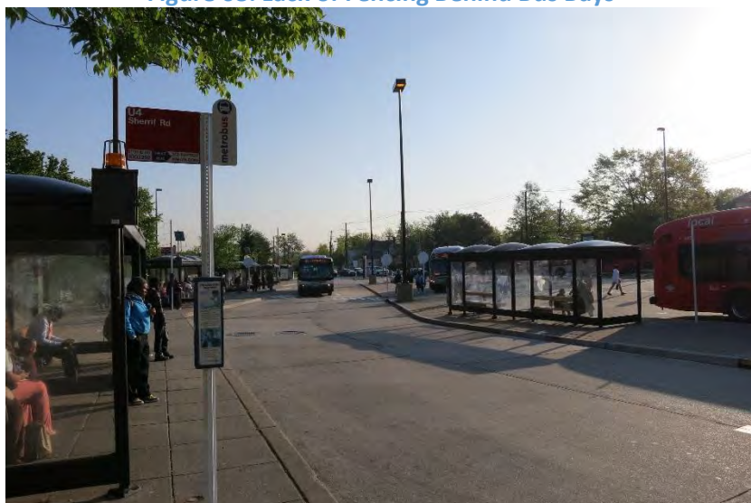
Figure 68: Lack of Fencing Behind Bus Bays
