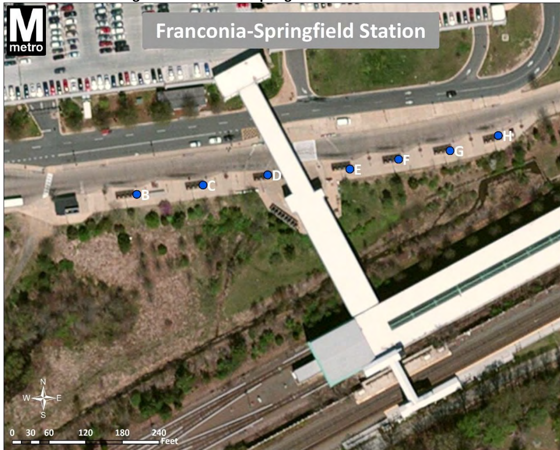
Figure 78: Franconia-Springfield Station Bus Shelters
