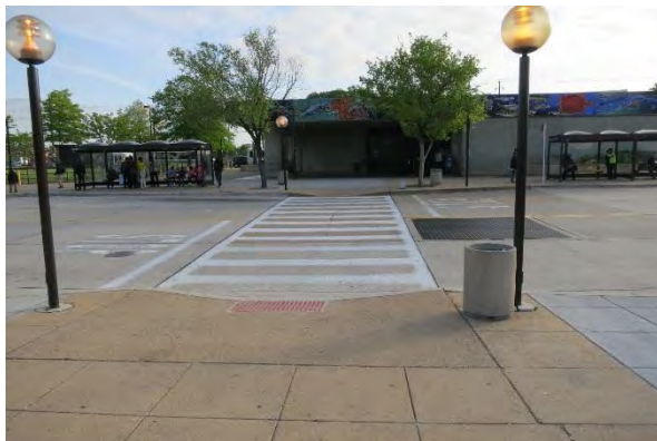
Figure 36: Main Busway and Crosswalk
