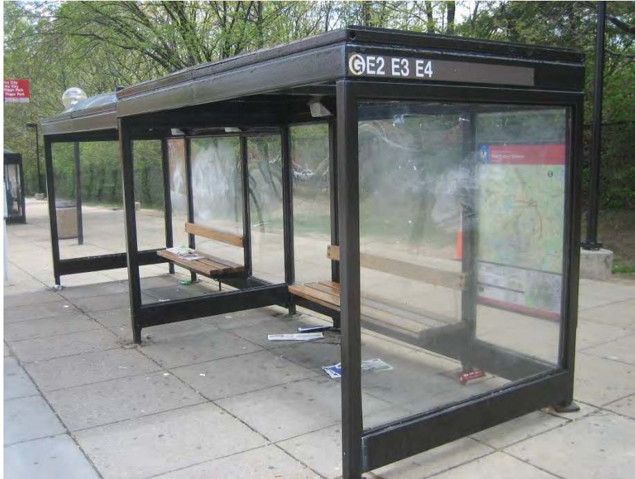
Figure 72: Poor Condition of Shelter G, Missing Panels, Rust and Missing Dome Top
