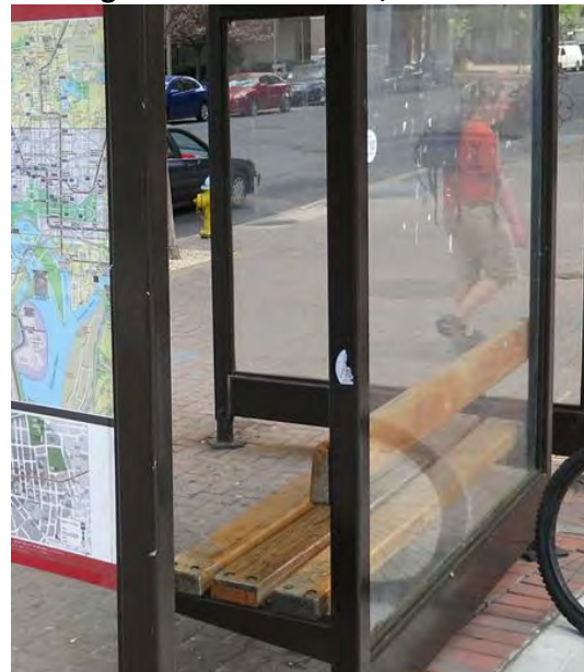
Figure 17: Worn Bench, Shelter H
