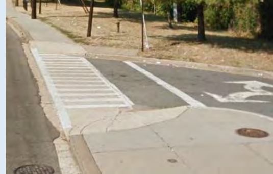
Curb Ramps at South Kiss-and-Ride Exit
