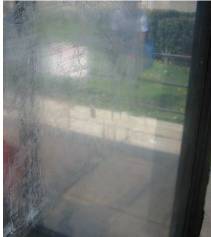
Figure 45: Smeared/Scratched Panel, Shelter E
