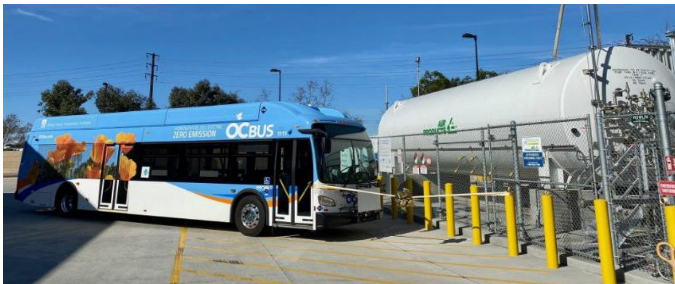
Figure 3-4. Orange County Transportation Authority's 18,000-Gallon Hydrogen Storage Tank
