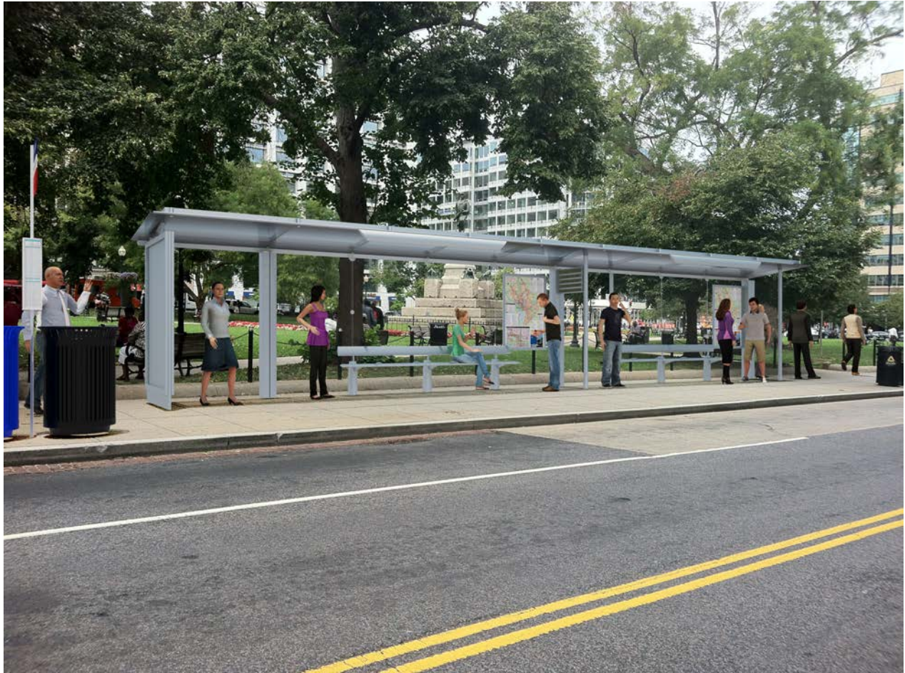
Figure 80: Custom-Sized Shelter at Stop 1001193 on Farragut Square
