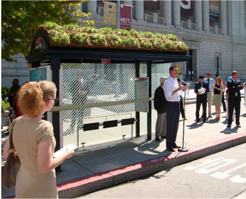
Figure 14: San Francisco Bus Shelter Green Roof Demonstration Project
