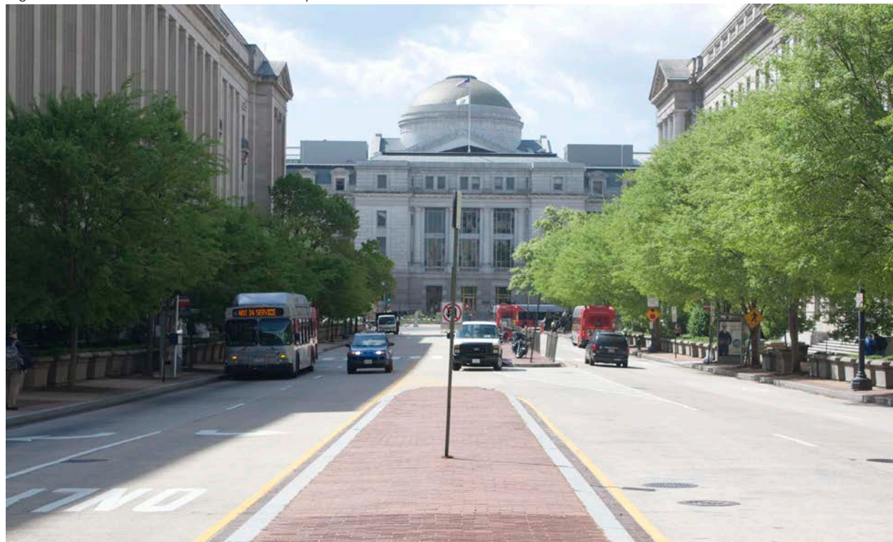
Figure 27: 10th Street NW between Pennsylvania and Constitution Avenues NW
