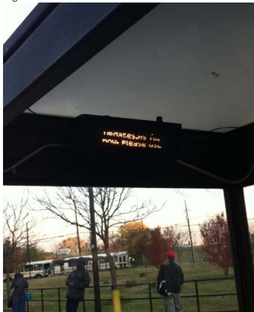
Figure 19: DMS at Anacostia Station
