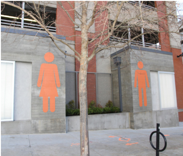
Market Square Garage, Knoxville, TN
