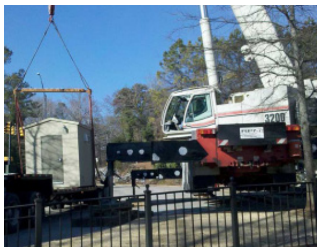
Prefabricated restroom crane installation
