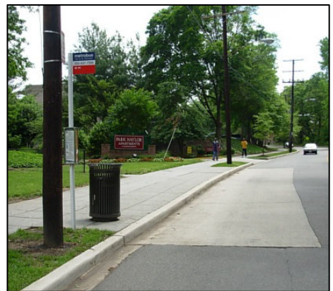
Expanded landing pad.
