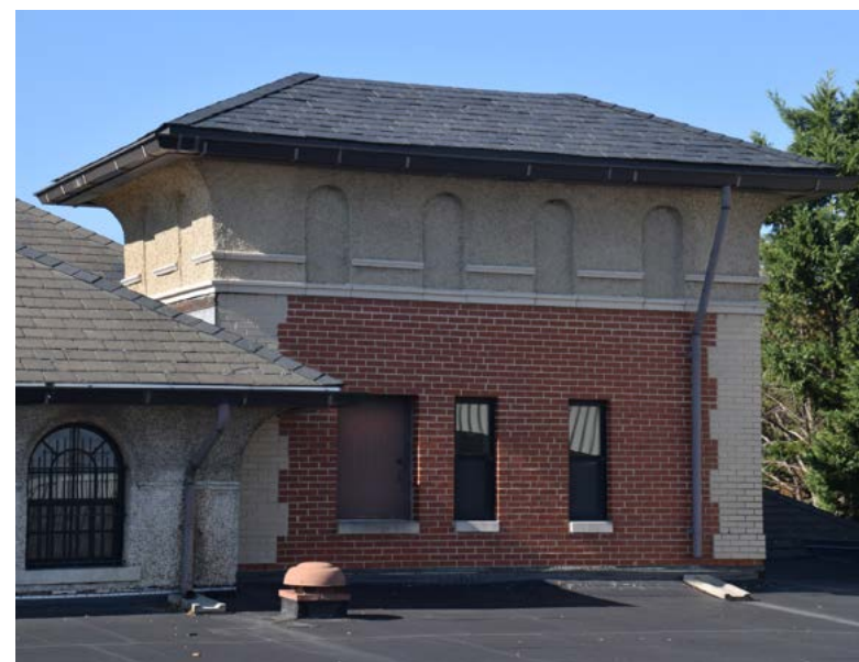
Non-historic stair and elevator tower, added 1987-1992
