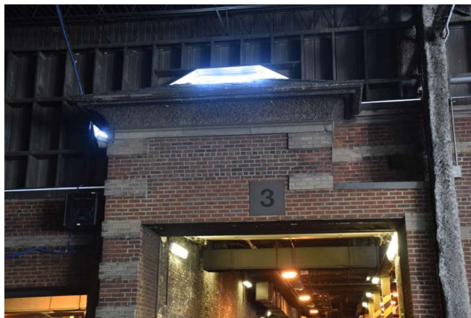
Hipped roof pavilion at north elevation
