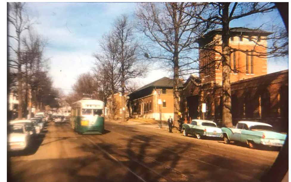
Car barn and tower, 1955-1962 (DC History Center)
