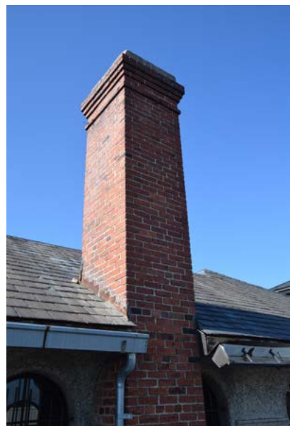
Admin offices chimney
