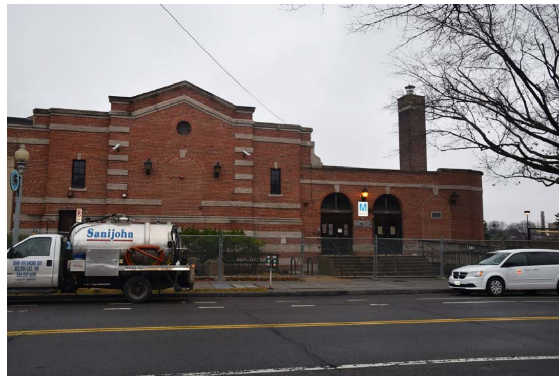
Southern end of west elevation; arched windows have been converted to door and window at center of pedimented bay has been infilled with brick
