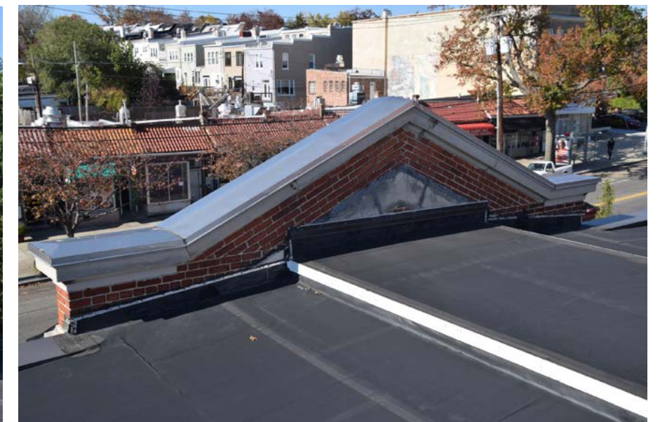
Triangular parapet facing 14th Street
