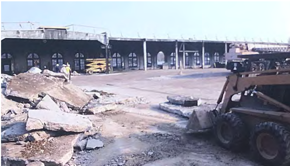
Figure 10. 1987 photograph looking east showing the extent of the demolition of ceiling and roof structure except for one bay along the perimeter of the east wall (WMATA Archive, George Washington University Special Collections)
