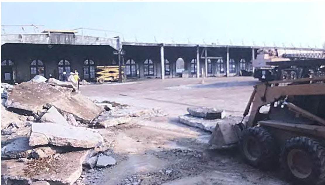
Figure 10. 1987 photograph looking east showing the extent of the demolition that occurred within the bus garage. The entire ceiling and roof structure in this area was removed except for one bay along the perimeter of the east wall (WMATA Archive, George Washington University Special Collections)
