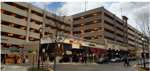
Dunn Loring Metro Transit Center
