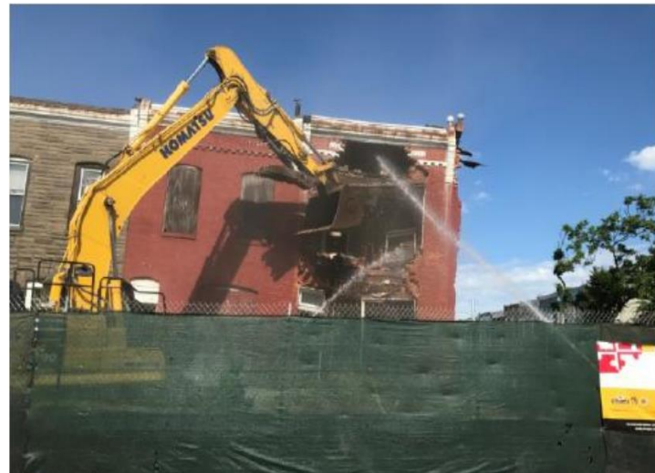
Maryland Stadium Authority – Project C.O.R.E.
