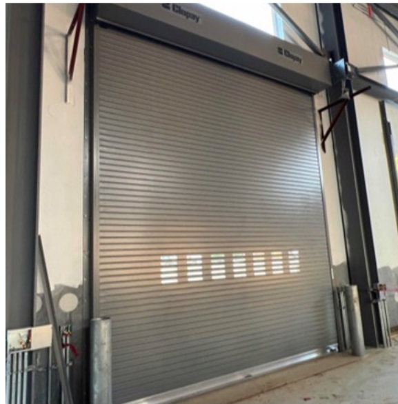
Overhead door install started
