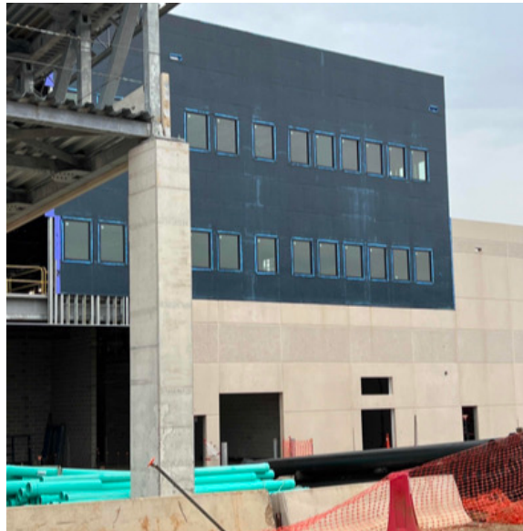
Glazing install ongoing
