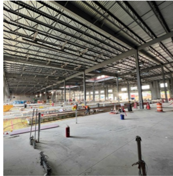
Slab on grade concrete ongoing
