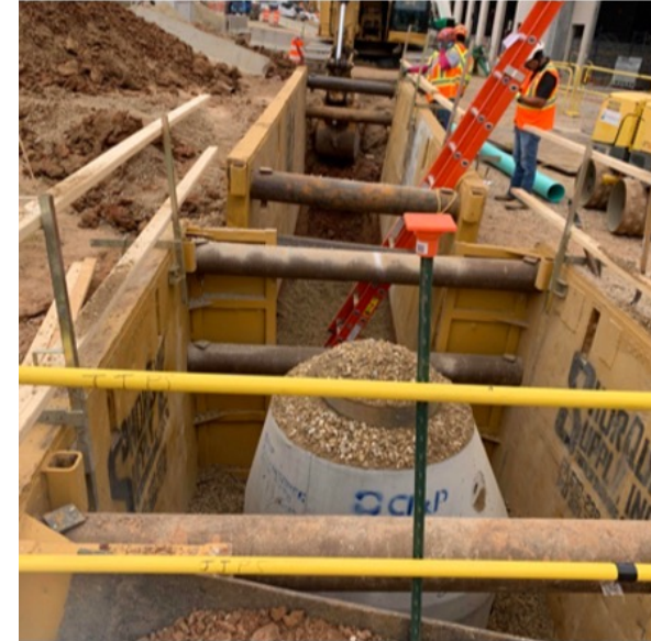
Site utilities started
