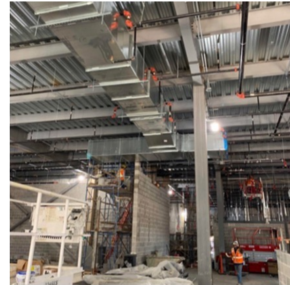
Overhead mechanical / electrical & plumbing ongoing
