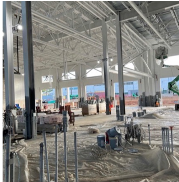
First coat of paint
