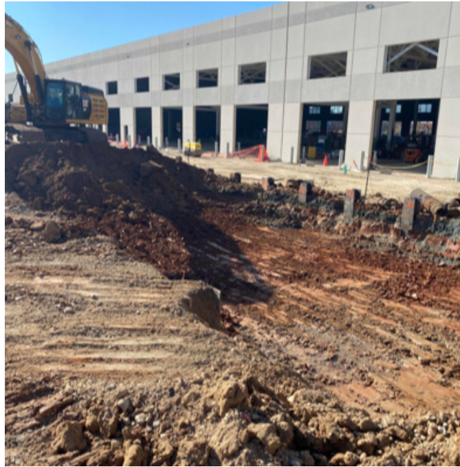
Start of Excavation
