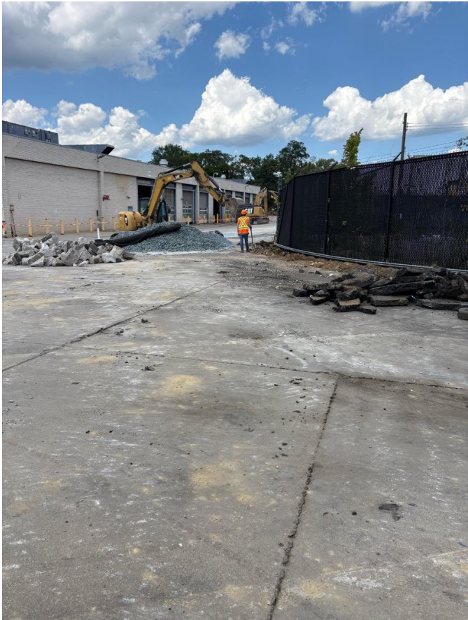
Stabilized Construction Entrance
