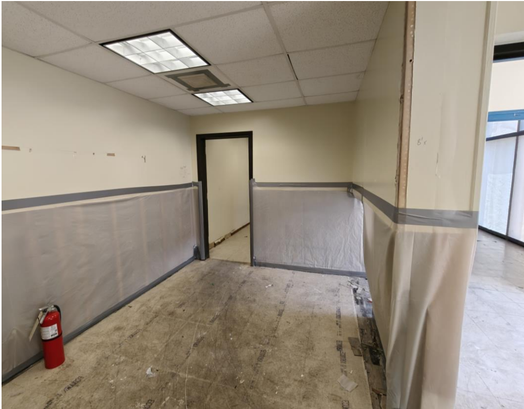
Ground Floor Abatement Preparation
