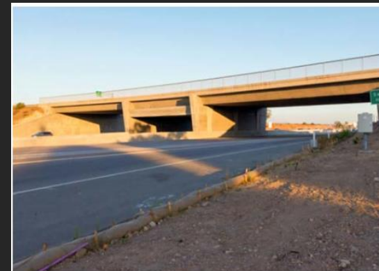
SAN DIEGO, CALIFORNIA, USA I-15 Express/BRT Lanes Improvement
