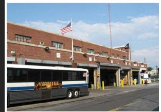
NEW YORK, NEW YORK, USA MTA Fleet and Facility Modernization
