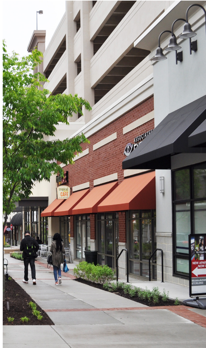
Figure 7.5 —Photograph showing integrated parking garage in joint development.
