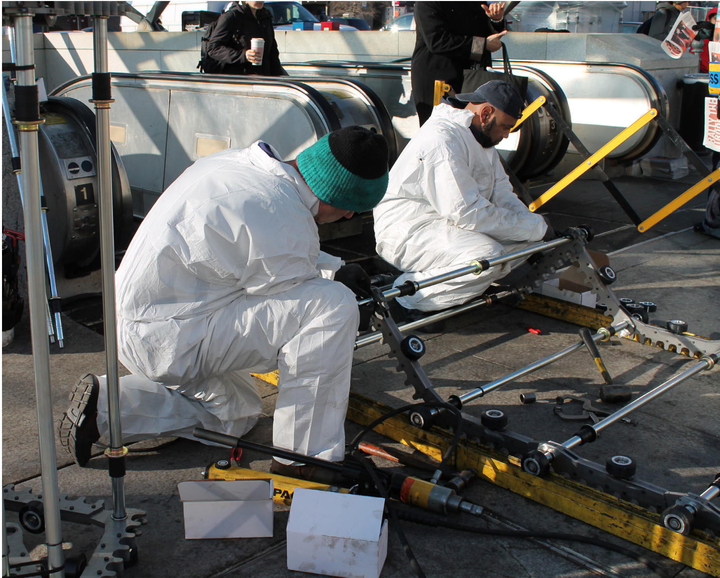
Figure 9.1 —Photograph of maintenance activities within station area. Elvert Barnes, FLICKR, https://creativecommons.org/licenses/by-sa/2.0/
