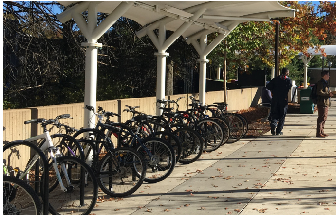
Example of U-Rack bicycle parking at Dunn Loring Metro Station.
