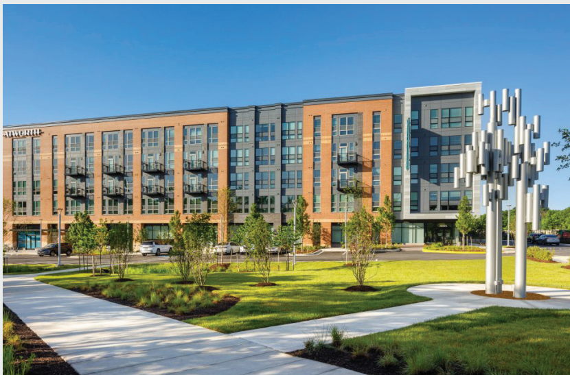
College Park—Atworth (Gilbane), 2024 451 units (100% affordable)
