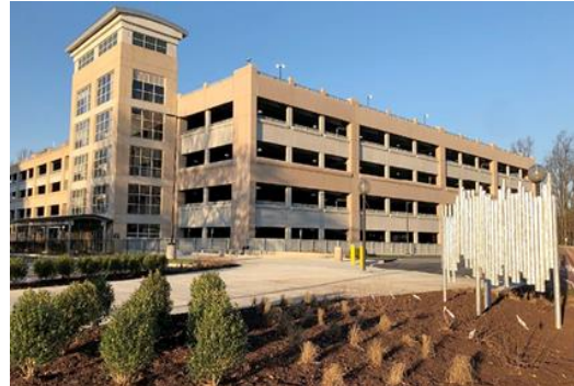
Passenger Parking Facilities
