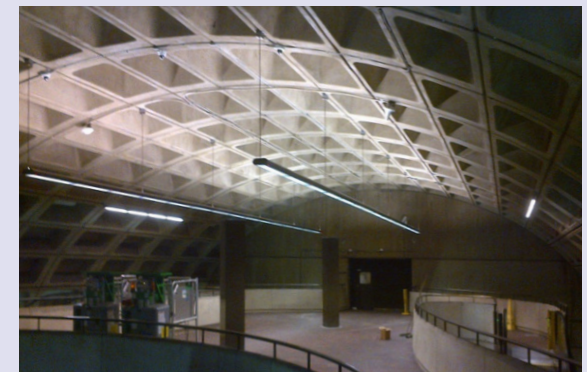
Improved station lighting permits a safer customer environment.
