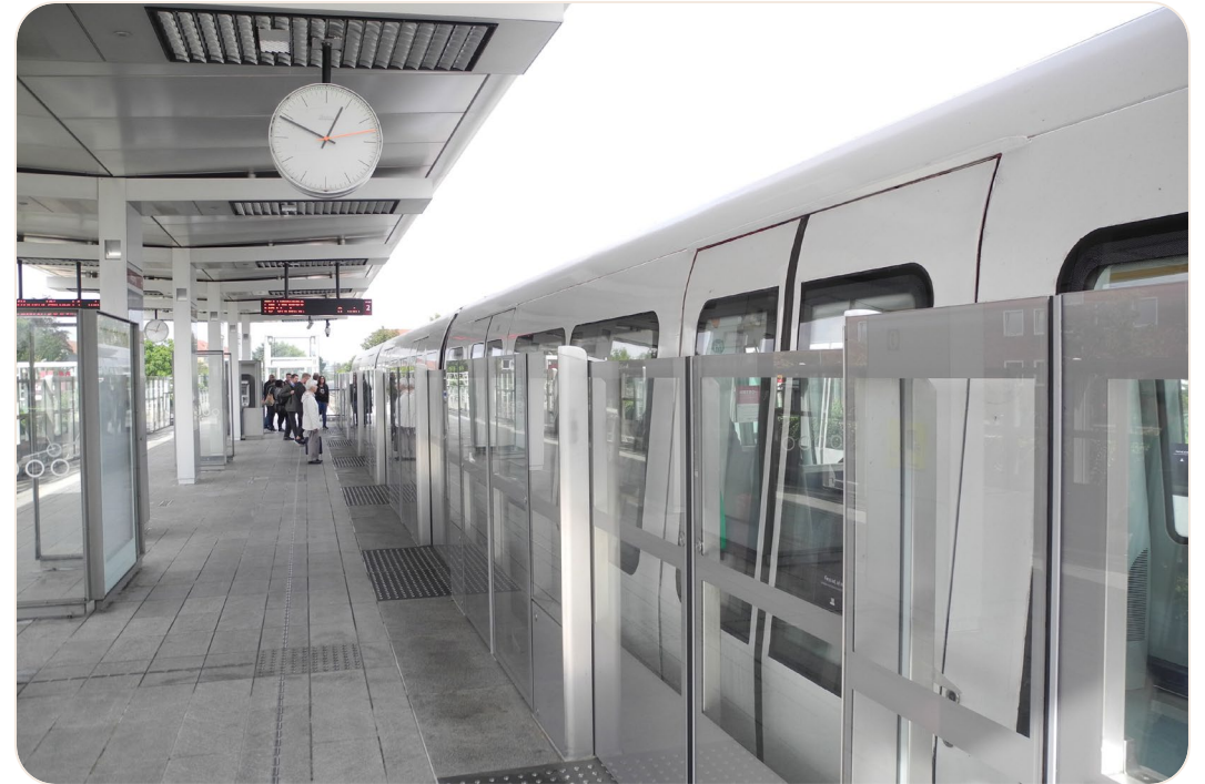
Kastrup Station, with platform screen doors – 2015
