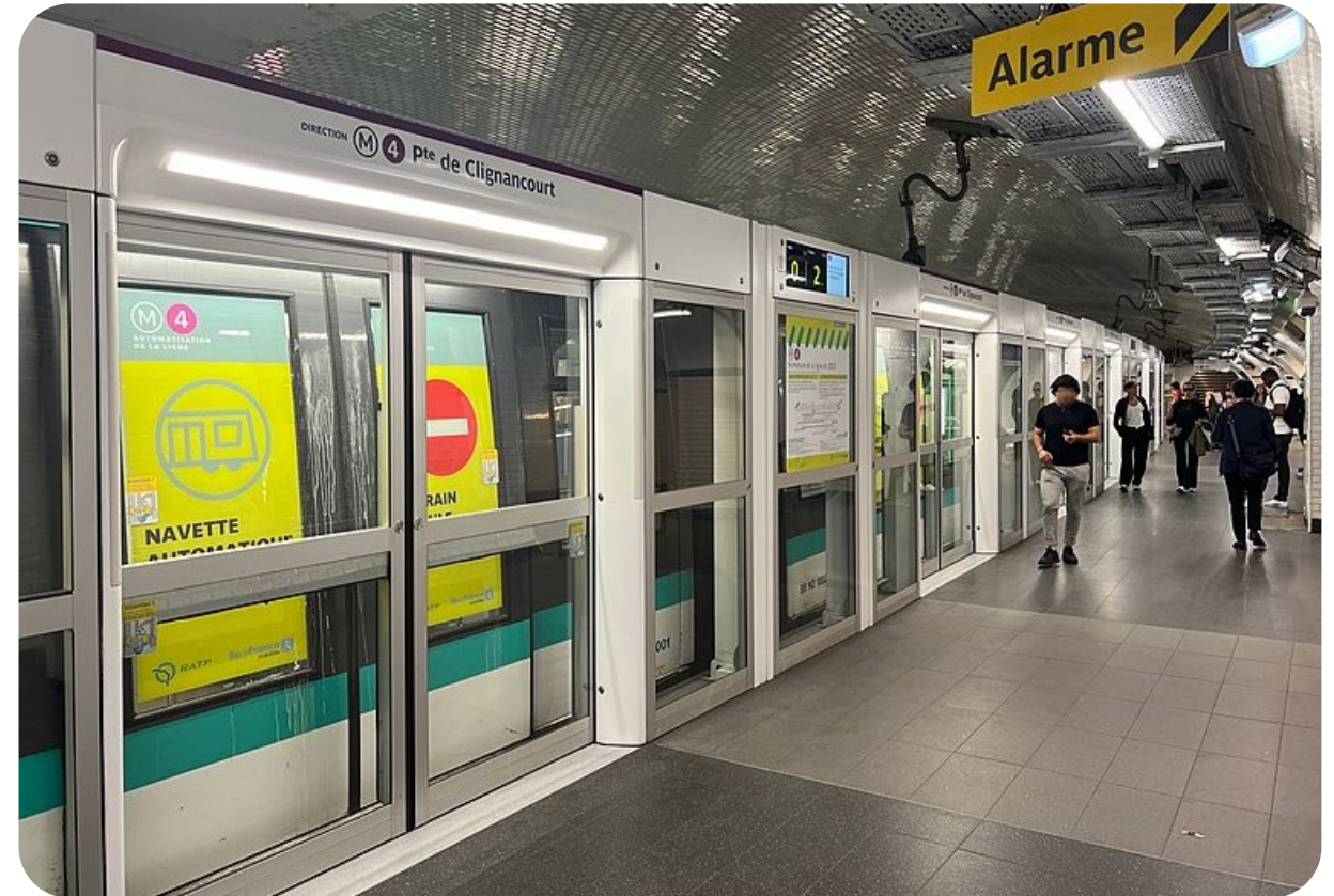
Paris Metro: Line 4 Platform Screen Door Testing
