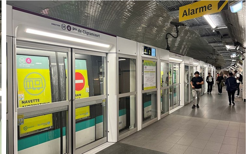
Paris Metro: Line 4 Platform Screen Door Testing
