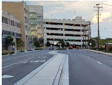
Figure 6: The Metro parking garage as viewed from Halpine Road and Rockville Pike.
