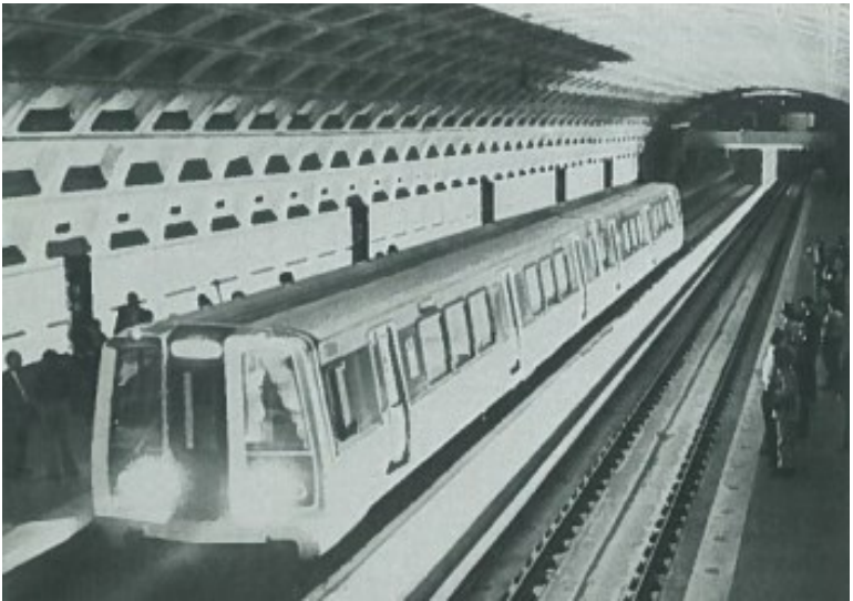
Metro was designed and built in the 1970s for automatic train operation (ATO) , which provides semi-automated operations.
