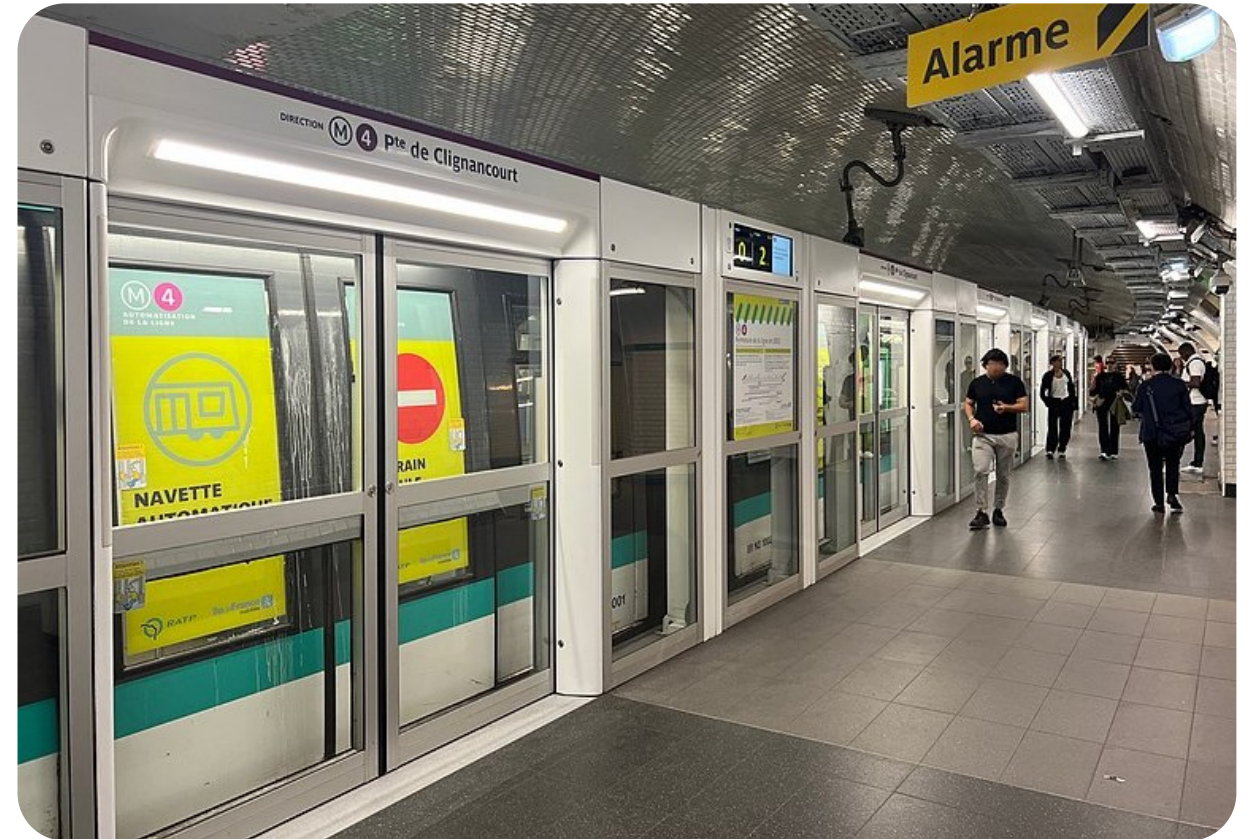
Paris Metro: Line 4 Platform Screen Door Testing
