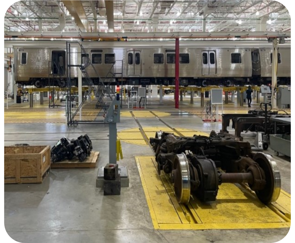
Dulles Yard Service & Inspection Building
