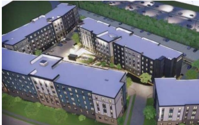
New Carrollton Phase 4 Groundbreaking (December) – Senior Living, 112 units (1 of 4 buildings, entire phase totals 364 units)
